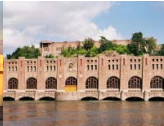
Olidan hydro power plant in Trollhättan.
