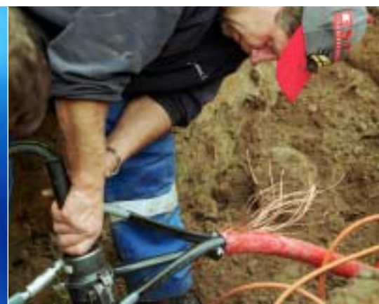
Joining an underground cable in Svenljunga.
