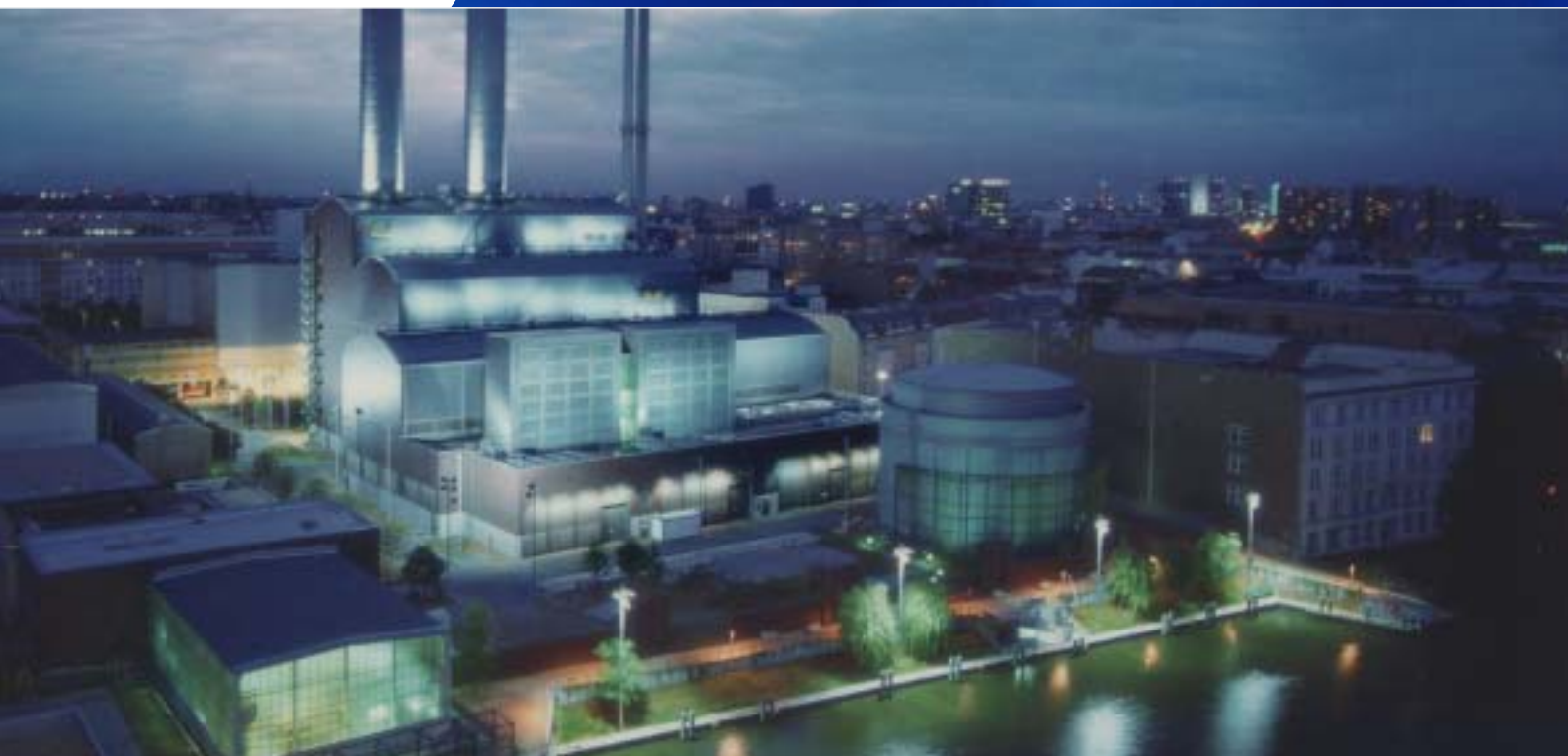
Thermal plant Mitte.
