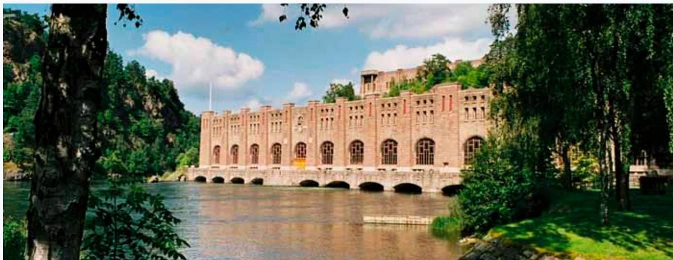
Olidan, on the Göta River, was one of the first hydro power stations built from 1909–1916 by the newly formed Swedish State Power Board.
