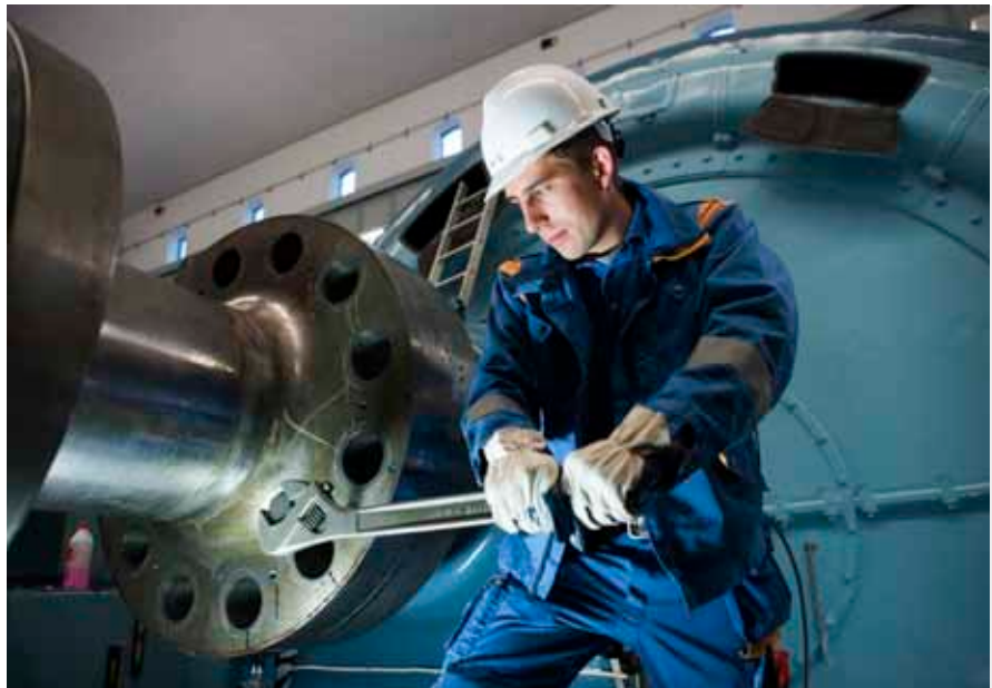
Maintenance work at the Älvkarleby hydro power plant in Sweden.
