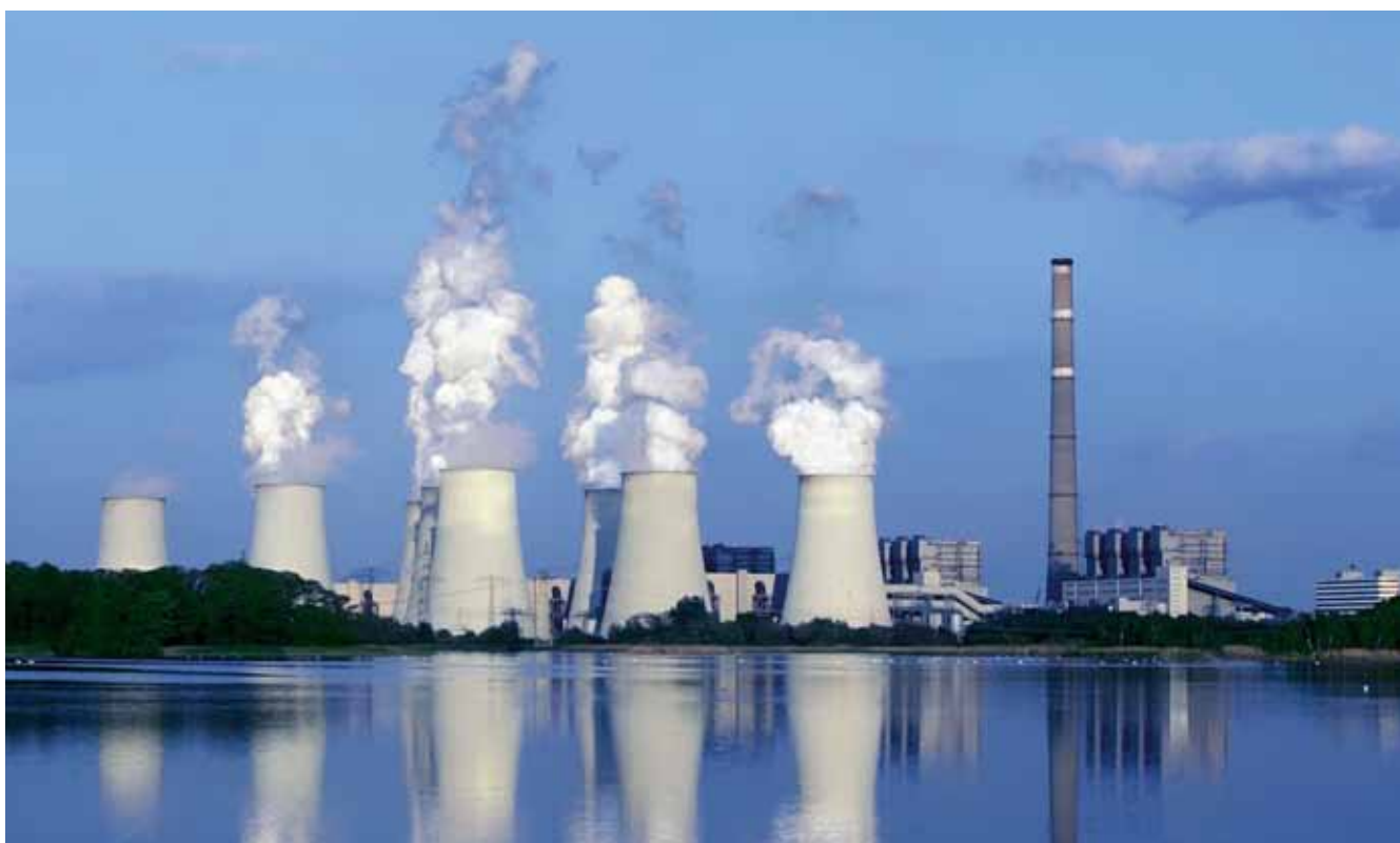
The Jämschwalde power plant in Germany.
