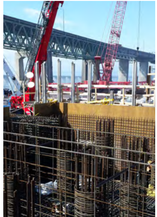
Samuel-De Champlain Bridge in Montreal (2016-2019)
