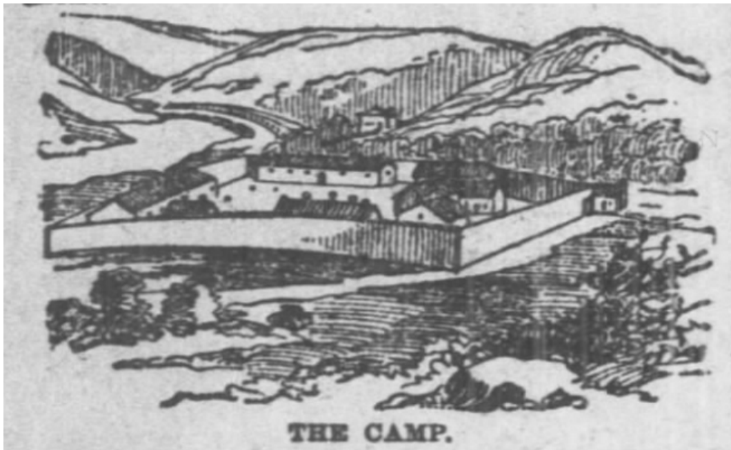
The above sketch is a depiction of the Stockade at Tracy City.
