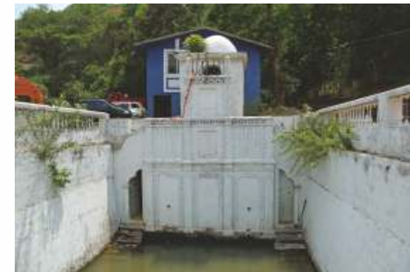
Fresh water spring at Mala
