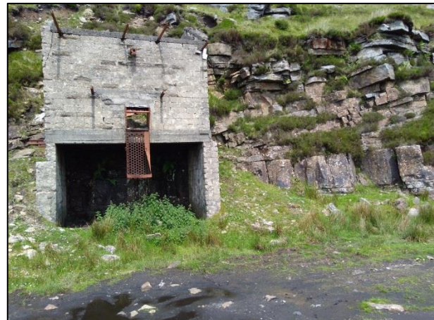
Screening plant, with cross-bedded sandstone units on right.
