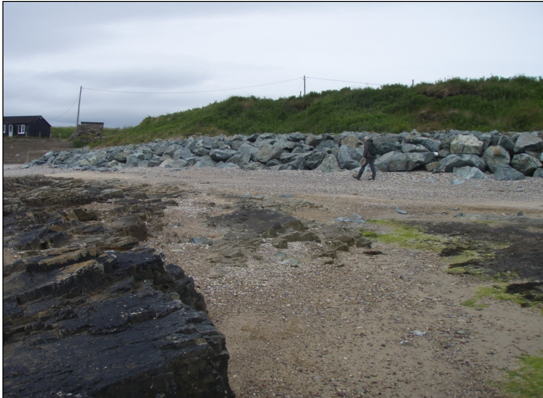
Coastal protection techniques include placing of large boulders at the toe of slumping areas, which are a significant modification of local landscapes. This photo of a boulder barrier is at Ballyquin.
