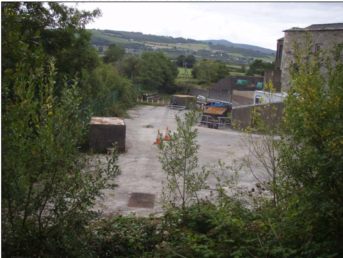
Four boreholes are contained in the yard at Ballynamuck West, underneath manhole covers.
