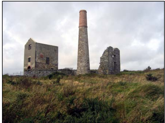
Tankardstown conserved mine buildings.
