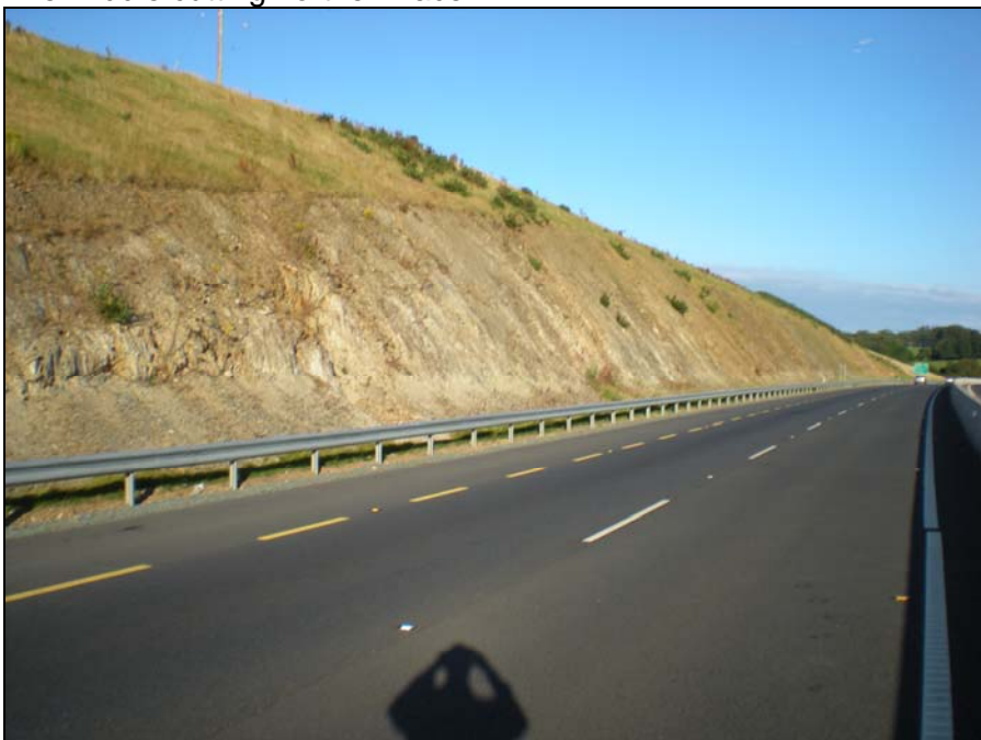
The western cutting, northern face, near the roundabout for Kilmeadan.
