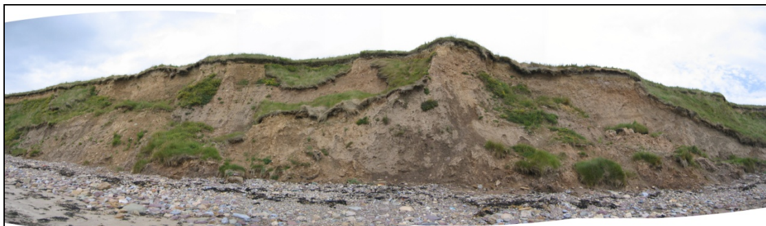
Slumps at Ballyquin Shore.
