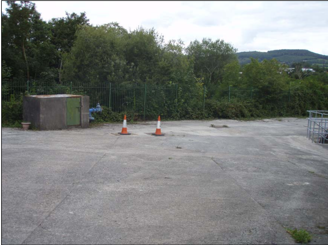
Two of the four boreholes are underneath the traffic cones.
