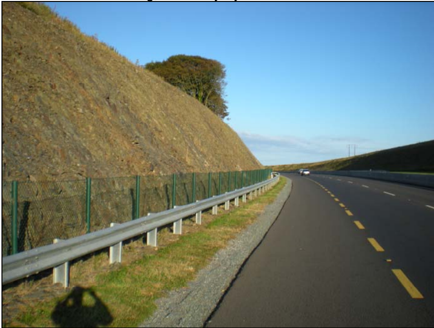
The middle cutting northern face.
