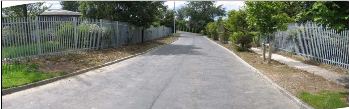
Panorama of the Cappoquin collapse of November 2010, picked out by the newly graded fresh earth in the road verges.
