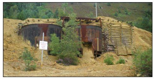
Ore bins installed in the late 1950s to hold ore trucked from the 850 adit and destined for the mill in West Avoca. One flatrod tunnel is located just to the right behind the bushes.
