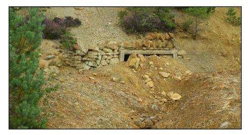
Timbered entrance to 850 Level adit partly hidden behind spoil. The channel in front was dug in recent years to accommodate a periodic discharge of water from the adit, a recent development possibly related to blocking of the normal drainage routes within the mine.
