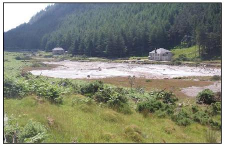
Area of tailings or fine waste material deposited downstream of the mine.
