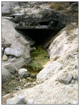
3<sup>rd</sup> Adit on Foxrock lode, July 2014, showing almost complete closure of entrance by siltation. Photo on right is from 2007.
