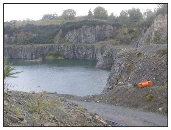
View southwards of western side of quarry, showing vertical faces and flooded quarry floor. Upper faces to right are readily accessible.
