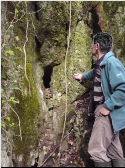
Conduit in Ballydoyle drive valley [168536 104600] note gravels at bottom of conduit (12/10/2009)
