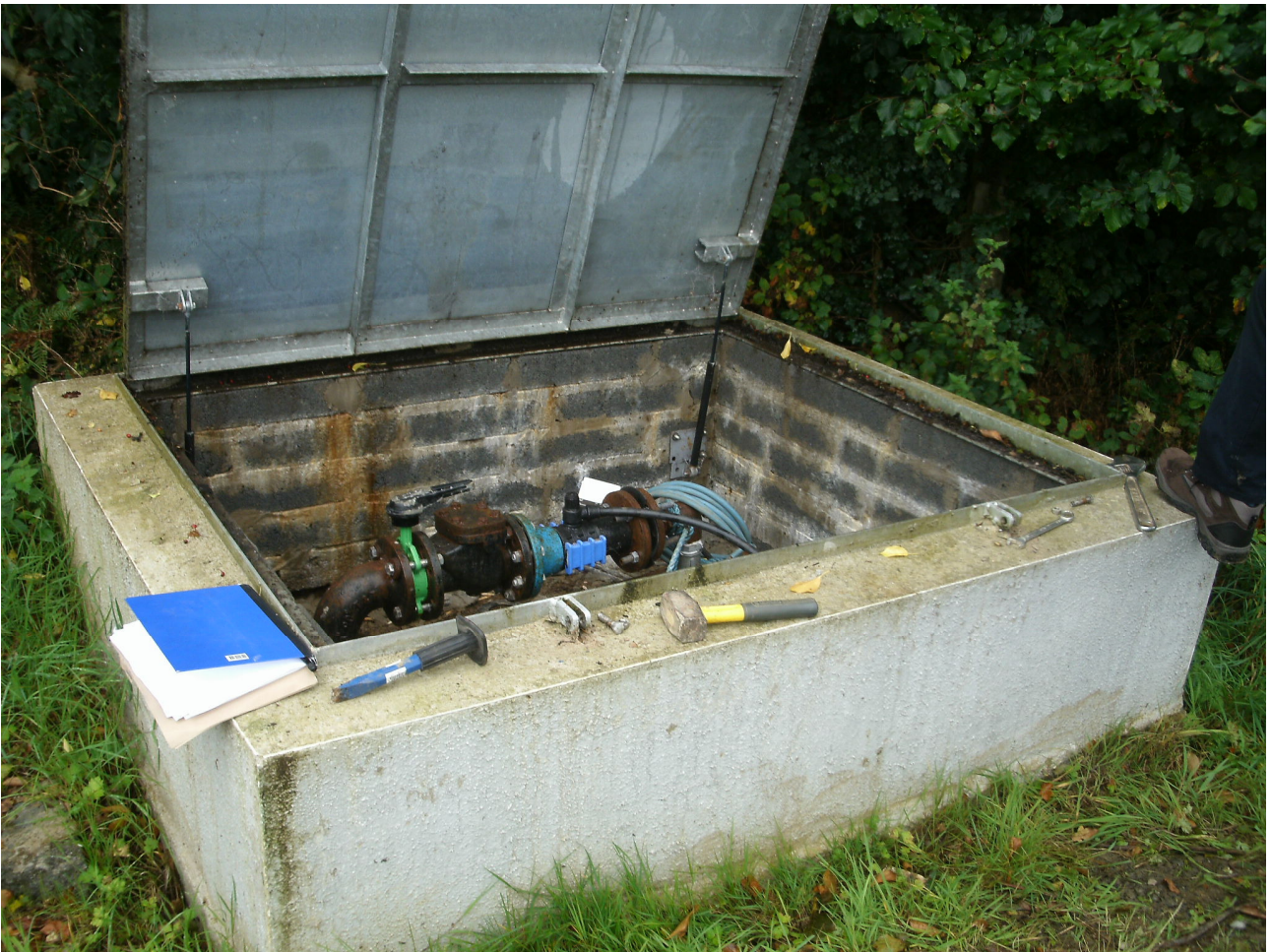
Photo 2 Concrete Chamber enclosing BH-1
