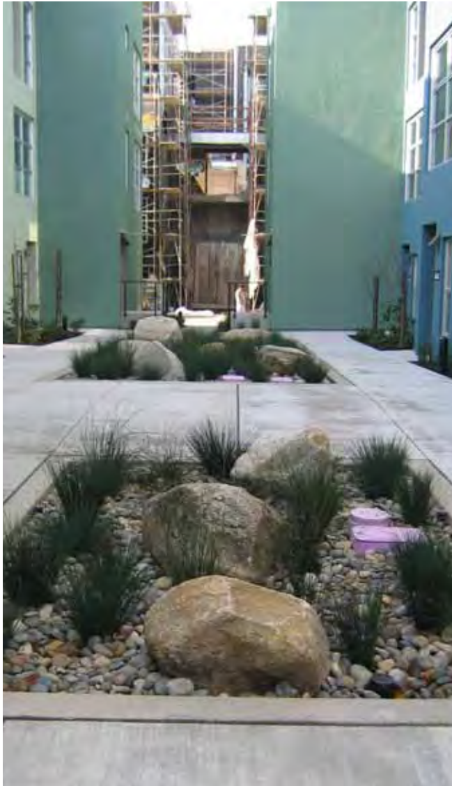
Linked bioretention cells are a central part of the design for the Glashaus development in Emeryville, CA.
