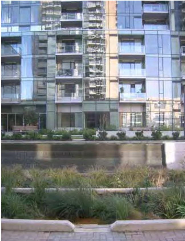
Stormwater treatment facilities enhance public spaces in Portland's South Waterfront redevelopment area.
