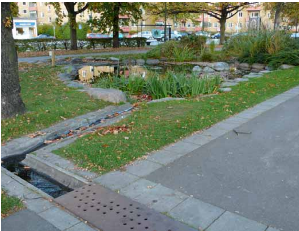
The Ekostaden residential development in Malmö, Sweden, channels all stormwater runoff through BMP treatment features such as bioswales, ponds, and wetlands as shown here. Photo: Brooke Ray Smith
