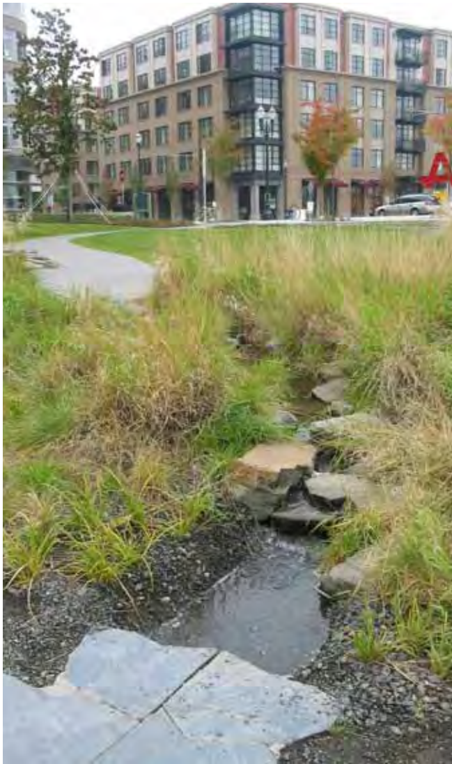
LID measures like the stormwater wetland in Portland's Tanner Springs Park treat polluted street runoff, thereby minimizing negative impacts to water quality.
