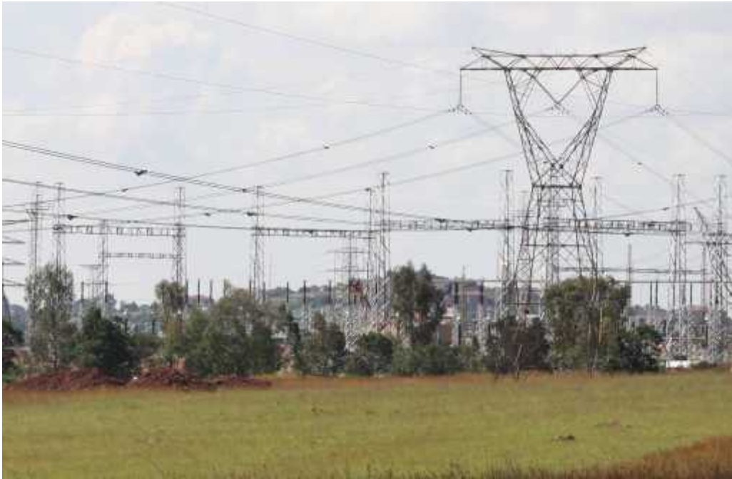
Photo 3 Doornkloof 129, view towards substation (north). Photo: February 2014, R.F. Terblanche.
