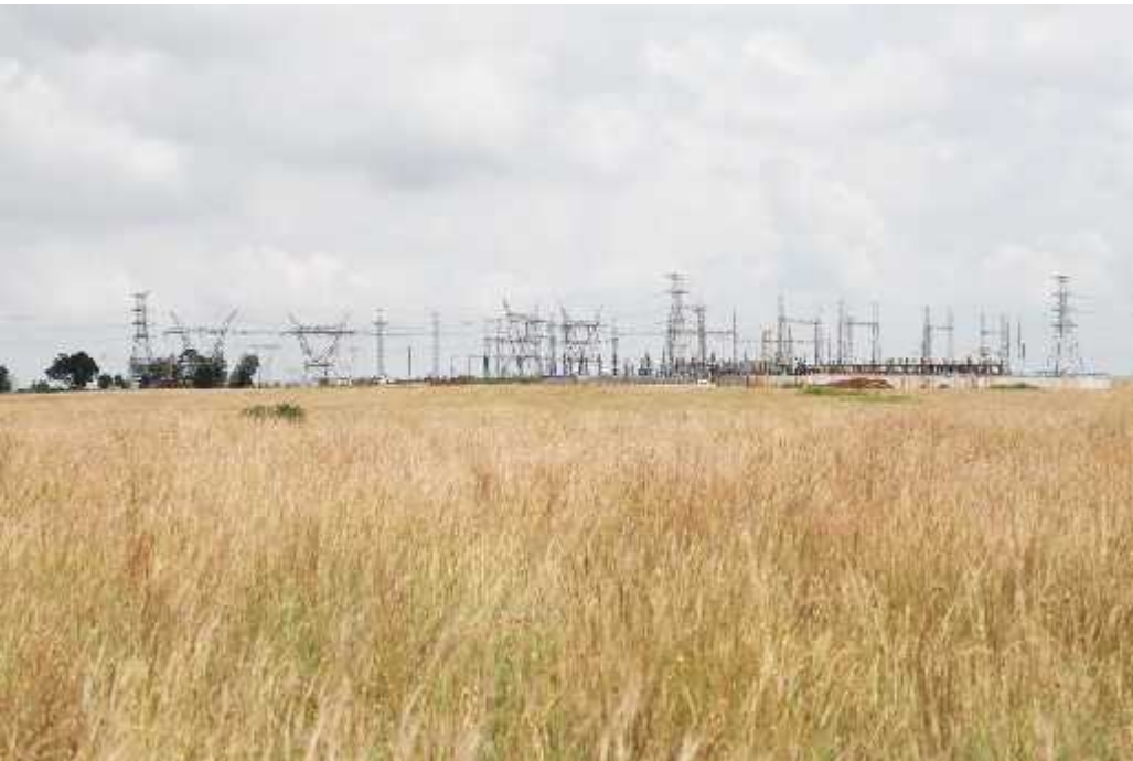
Photo 2 Doornkloof 107, view towards substation (to the south). Photo: 22 February 2014, R.F. Terblanche.
