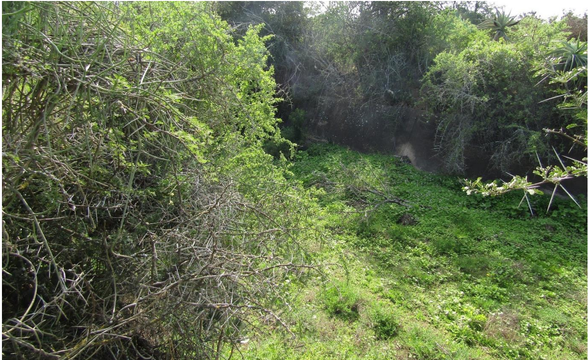
2.5. Example of the old concrete canal, overgrown here with alien and weedy species, and generally lined with Vachellia (Acacia) karroo .
