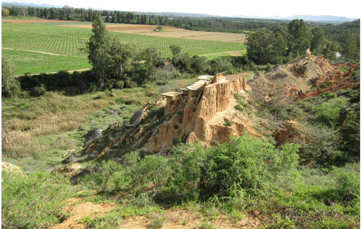
1.5. Photograph of severe erosion on the steep slopes above the Sundays River (at the northern end of the property). Note the old concrete canal, which is broken.
