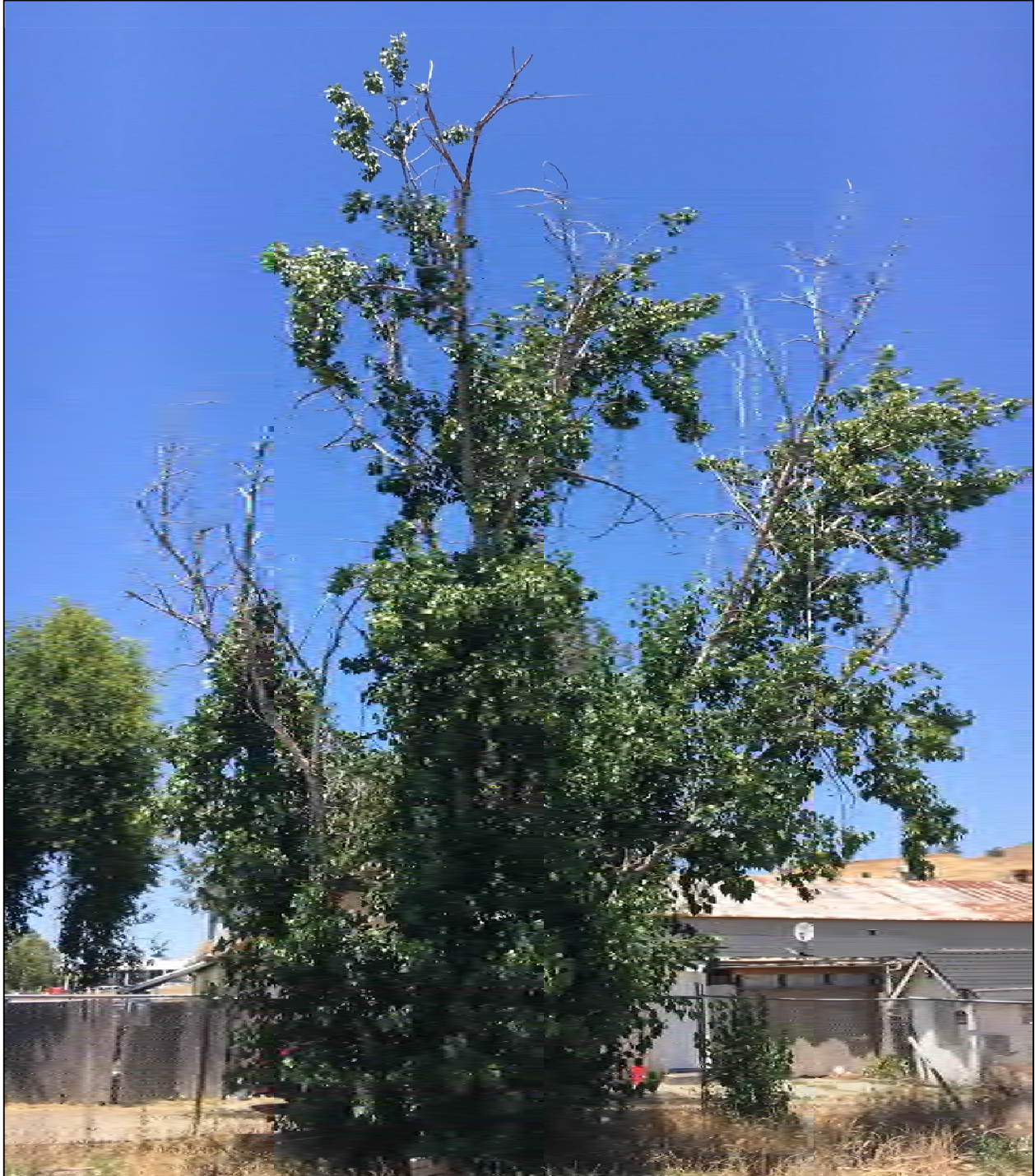
Photograph 4. Photograph depicting protected tree #625, an overmature, declining, multi-trunk black poplar tree. This tree was assessed in poor health and structure due to presence of multiple trunks with included bark and significant dieback of major trunks and scaffold branches. The appraised value was determined to be $890.
