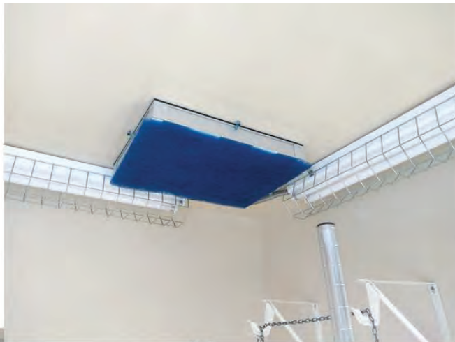
HEPA Filters (with blue pre-filters) installed over exhaust vent on Feb 11 2020
