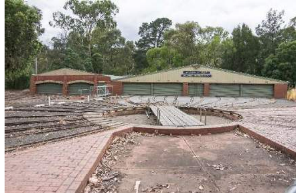
Figure 13. The turntable in the foreground. (Source: Context 2020)
