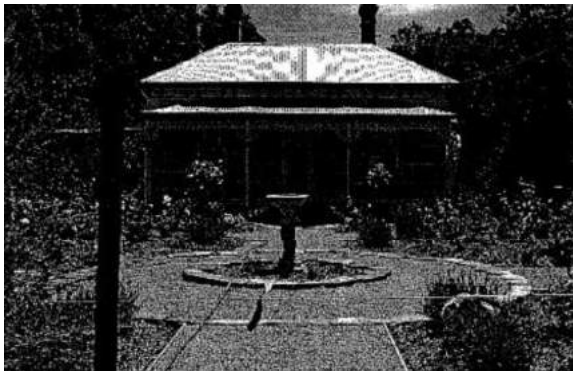
Cracknell orchard house, 395-405 Kangaroo Ground-St Andrews Road, Panton Hill (HO221). (Source: VHD)
