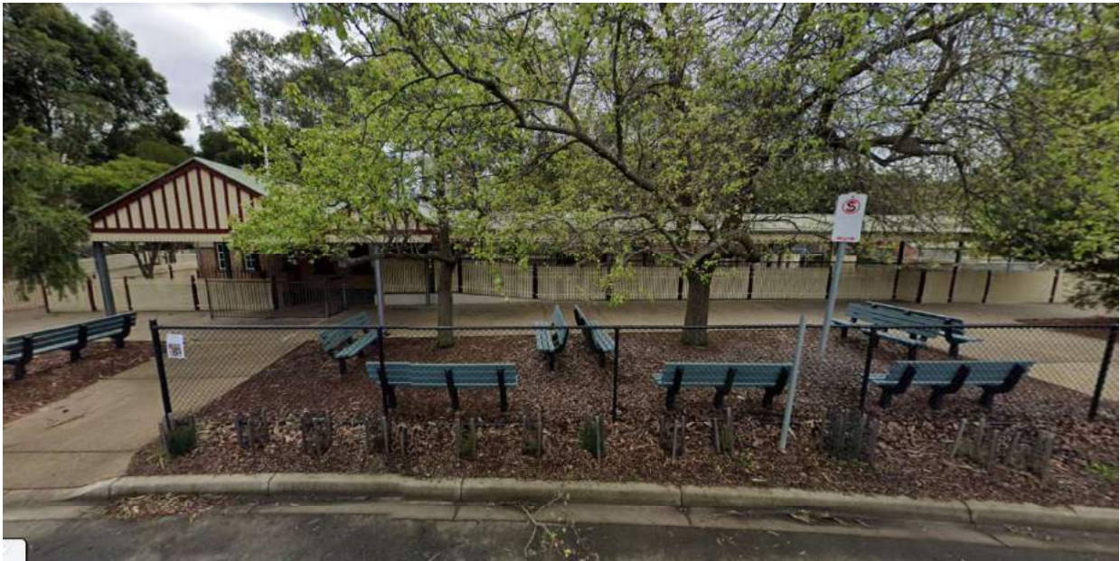
Figure 4. Primary entrance to the Main Station building (southwest elevation). (Source: Google Streetview 2019)
