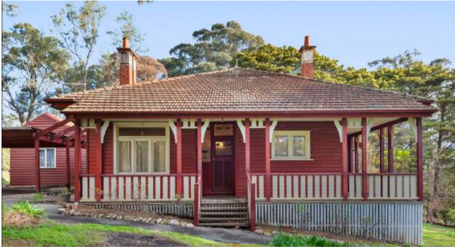
Figure 5. Principal (northeast) elevation 1080 Heidelberg-Kinglake Road, Hurstbridge. (Source: realestate.com.au 2019)
