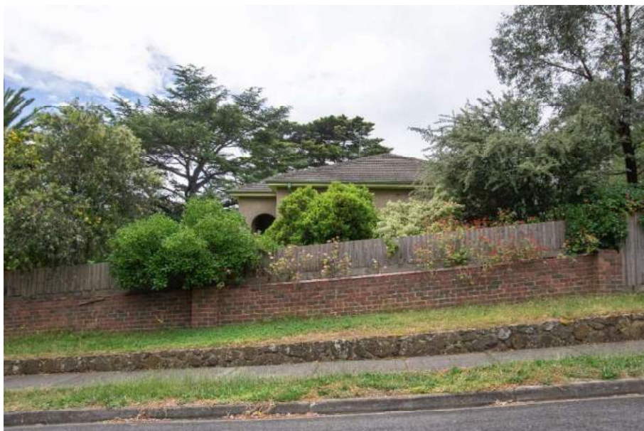
Figure 2. 2 Batman Road, Eltham, secondary elevation from Livingstone Road. (Source: Context 2020)
