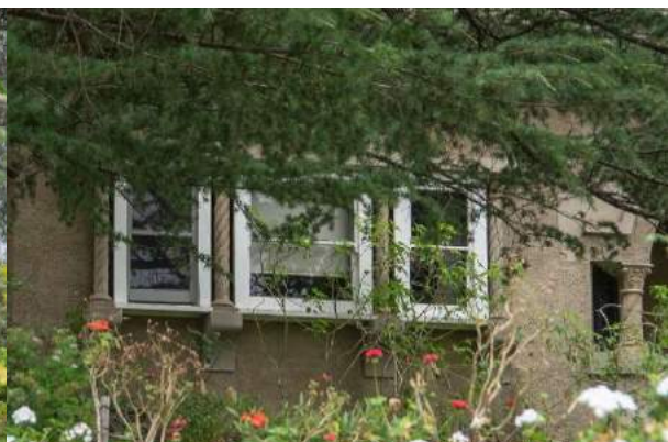
Figure 13. Windows separated by barley twist mullions atop smooth corbels. (Source: Context 2020)
