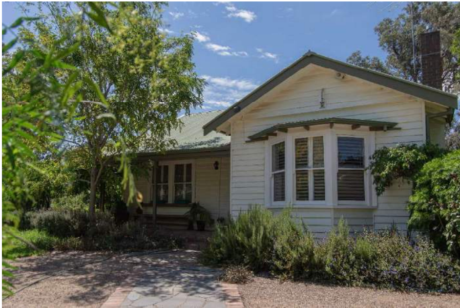
Figure 1. 200 Ryans Road, Eltham North, viewed from the west. (Source: Context, March 2021)
