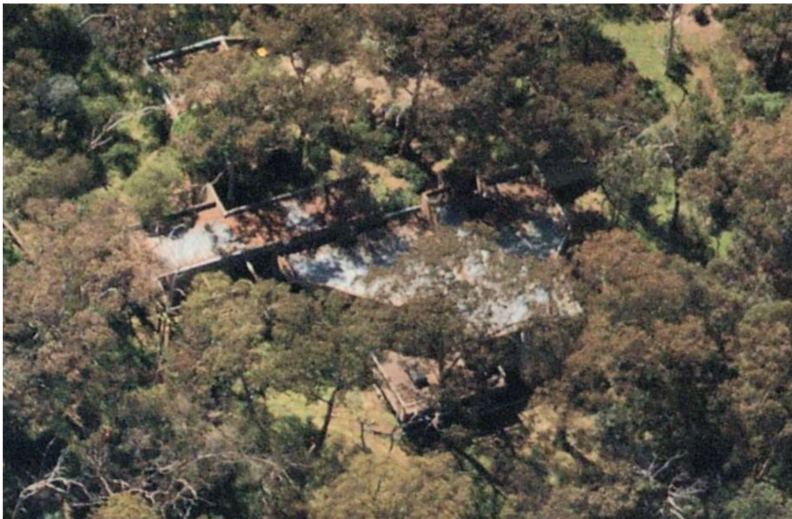
Figure 9. Aerial view looking east showing the carport at the top of the block, single storey wing of interconnecting cubes towards the middle and rear lower portion of the house angled to the north and leading onto an open timber deck. (Source: Nearmap 2020)
