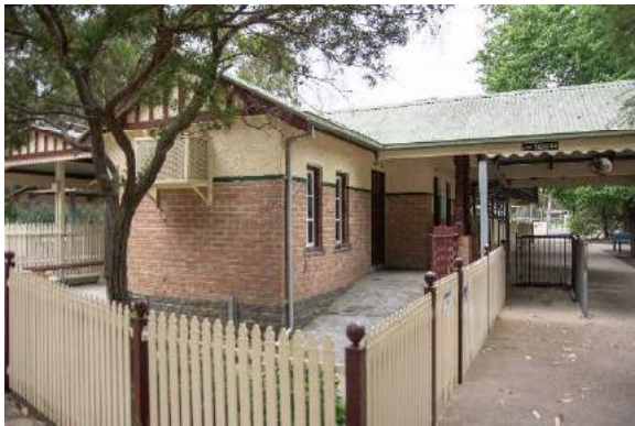
Figure 6. Station building with scalloped fascia. (Context 2020)
