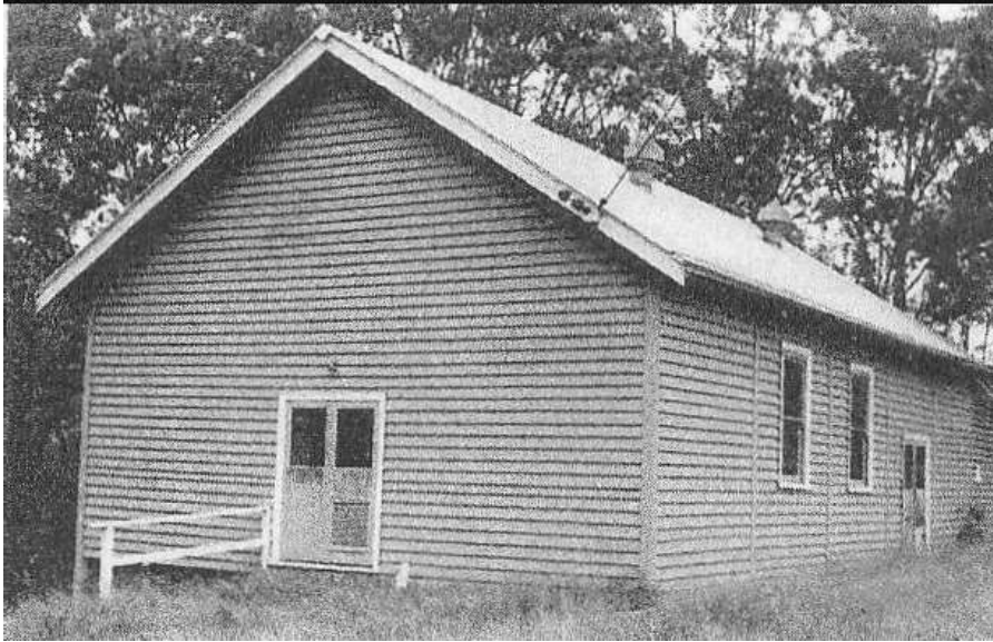
Figure 3. St Andrews Hall, c1965. (Source: Reynolds nd)
