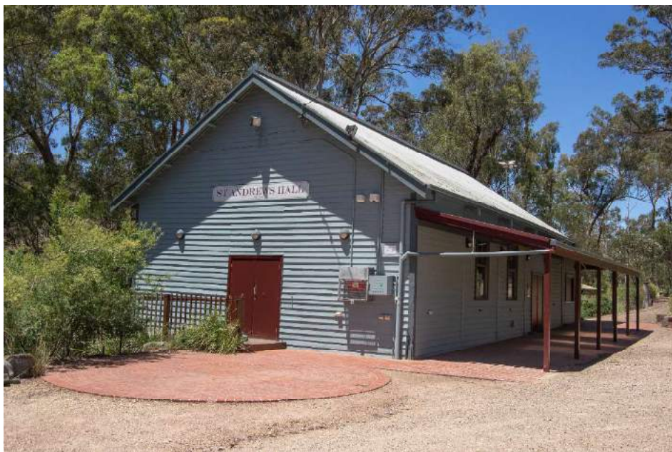
Figure 2. The northern end of St Andrews Hall. (Source: Context 2020)
