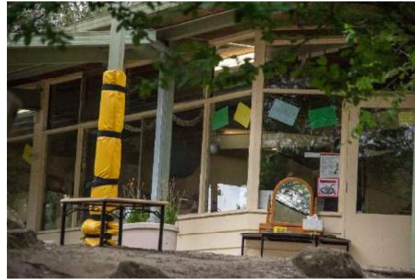
Figure 19. Window wall at the southern corner of the southern façade. (Source: Context 2020)
