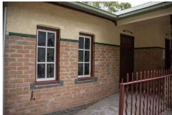
Figure 9. Six paned timber framed windows and decorative fence. (Source: Context 2020)
