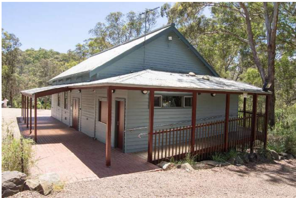
Figure 1. The southern end of St Andrews Hall. (Source: Context 2020)
