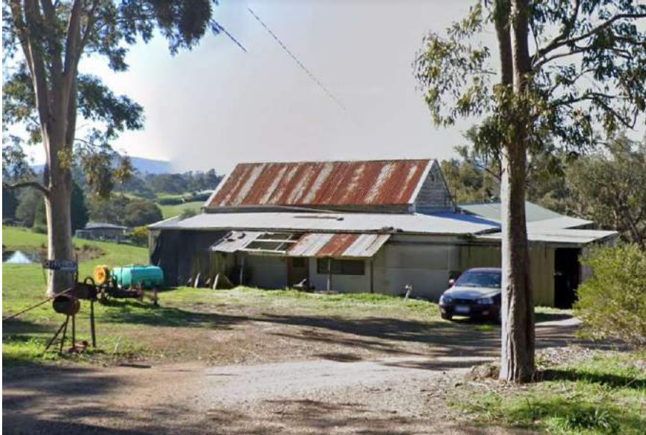
Figure 21. The primary (south) elevation of 191 Cherry Tree Road, with an attached garage, replaced window and door joineries and extended verandah. (Source: Google 2019)
