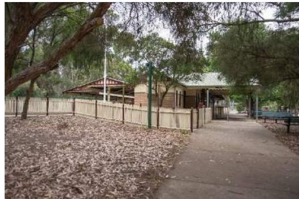
Figure 7. View of the station from the northwest. (Source: Context 2020)
