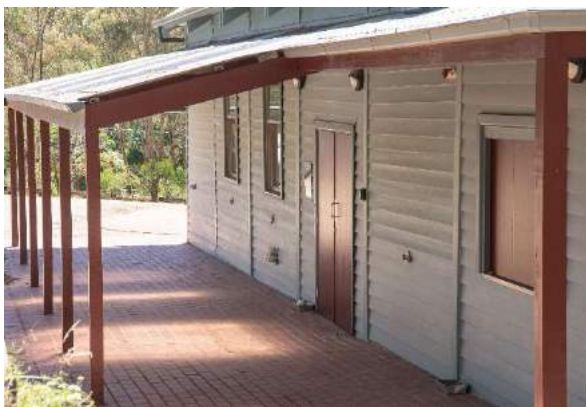
Figure 10. Corrugated iron verandah supported by timber posts over red brick paving. (Source: Context 2020)
