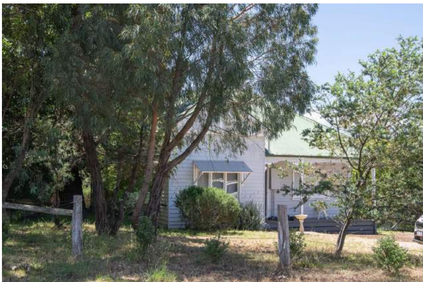
Figure 2. 173 Cherry Tree Road, Hurstbridge. (Source: Context 2020)
