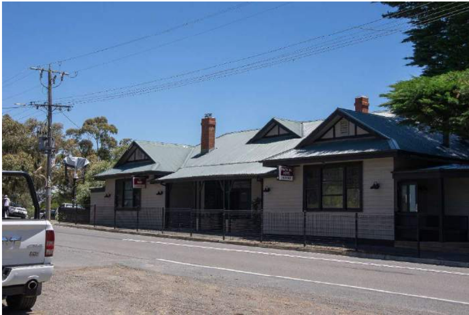
Figure 1. Panton Hill Hotel from St Andrew-Kangaroo Ground Road. (Source: Context 2020)
