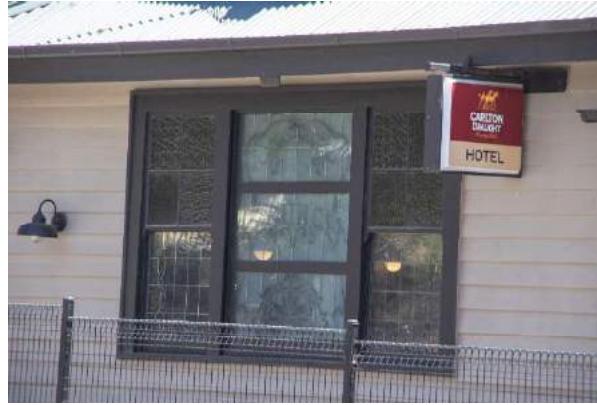
Figure 14. Tripartite bay window with ledlight and textured glass glazing. (Source: Context 2020)
