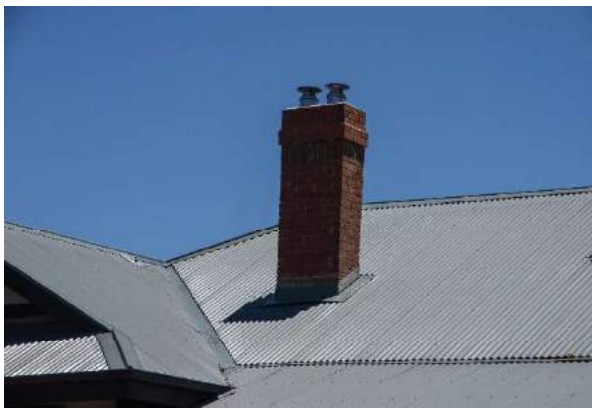
Figure 15. Brick chimney extending through the roof plane. (Source: Context 2020)
