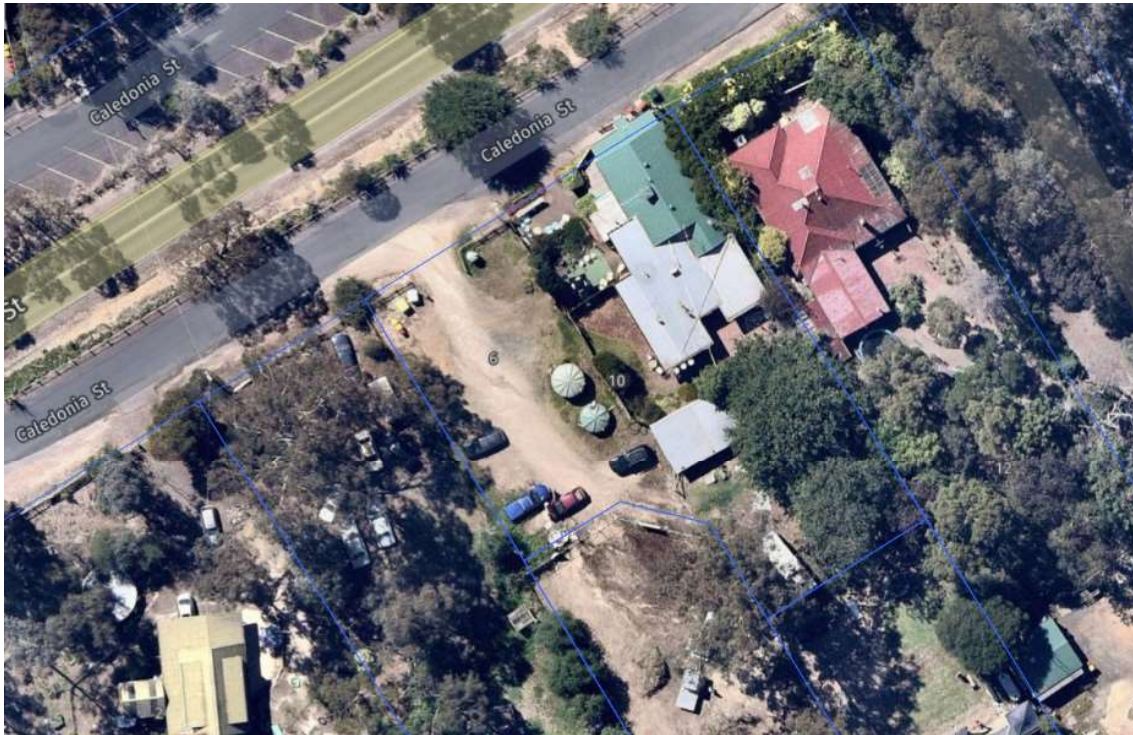
Figure 6. Aerial imagery of the site. (Source: Nearthmap 2021)
