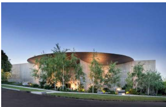
Towers Road House, 9 Towers Road Toorak, Stonnington City (Source: Wood Marsh)
