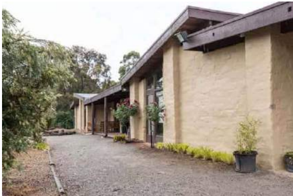
Coller House, 185 Mount Pleasant Road, Eltham (HO136). (Source: T Knox nd)
