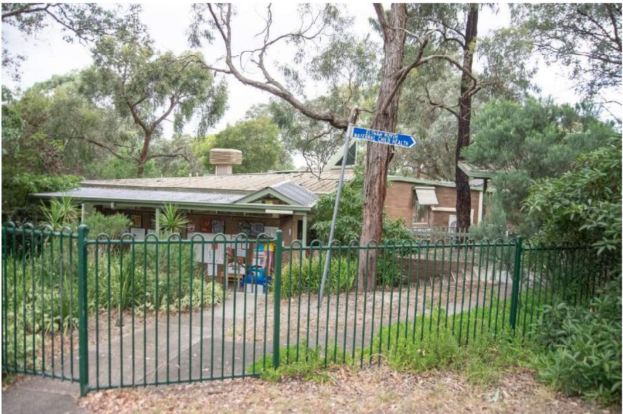
Figure 9. The entrance to the Preschool from the carpark showing the pathways to both pavilions and concrete stairs behind the aluminium fence. (Source: Context 2020)
