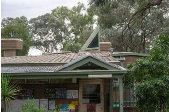
Figure 14. Small gable at main preschool entrance set above a skillion roofed verandah extension clad in corrugated iron. (Source: Context 2020)
