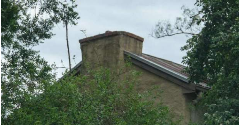
Figure 14. The mudbrick chimney of the study. (Source: Context 2020)
