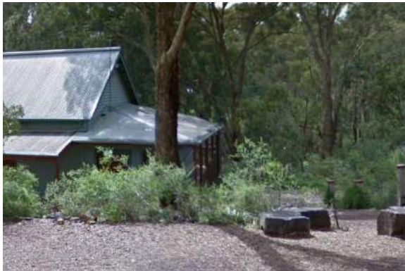
Figure 8. Kitchen addition to the rear of the building. (Source: Google Streetview 2016)
