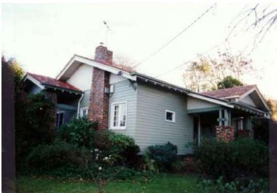
149 Mt Dandenong Road, Croydon (HO105, Maroondah City). (Source: VHD)
