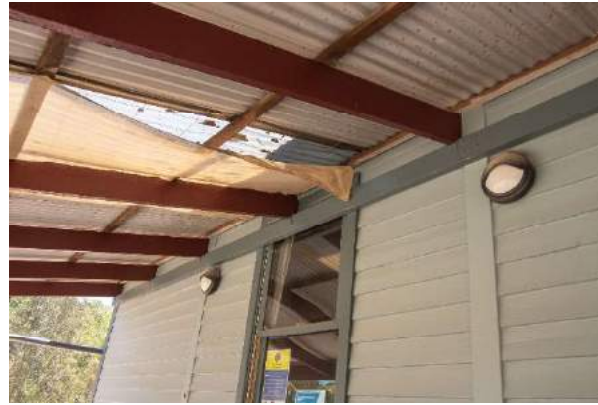
Figure 13. Window, corrugated iron and translucent polycarbonate clad verandah. (Source: Context 2020)
