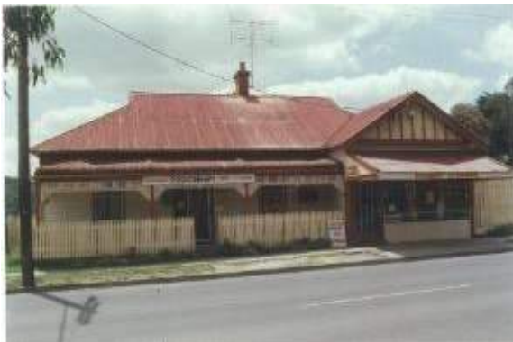
Former Butcher's Shop and House, 919 Heidelberg-Kinglake Road, Hurstbridge (HO75). (Source: VHD)
