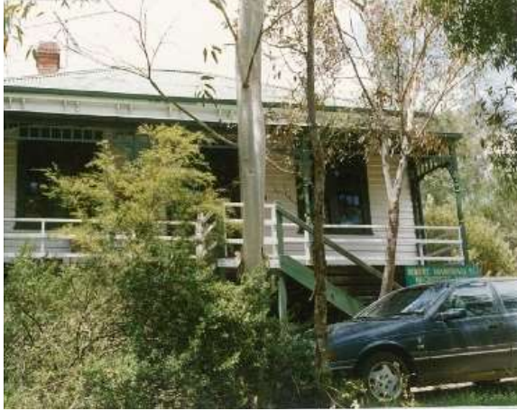
'Daraville', 828 Heidelberg-Kinglake Road, Hurstbridge (HO70). (Source: VHD)
