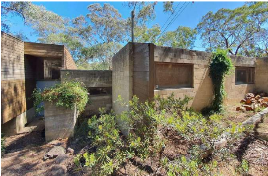
Figure 2. The principal elevation of 14-16 Warringah Crescent, Eltham, looking north-easterly. (Source: Context 2021)
