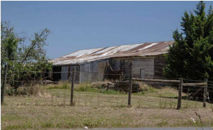
Figure 1. The cool store at 180 Cherry Tree Road, Hurstbridge, viewed from the northeast. (Source: Context 2020)
