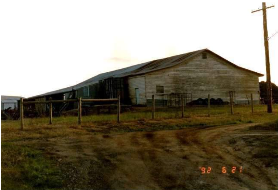
Figure 6. Cool shed at 180 Cherry Tree Road in 1992, viewed from the northwest (upper) and the northeast (lower). (Source: VHD)
