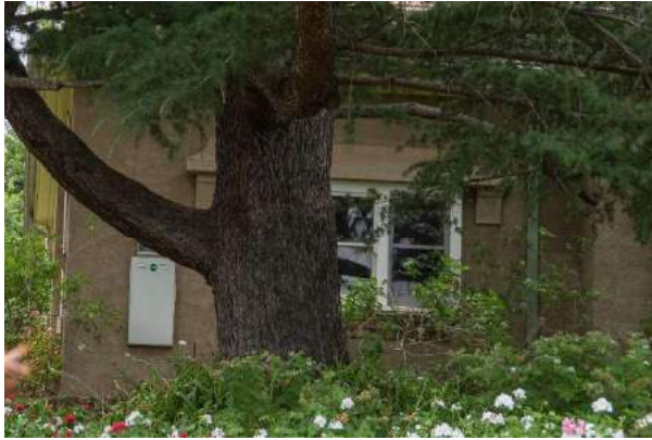
Figure 14. Second tier window detailing, with stepped brick sills and broad smooth rendered lintel supported by corbels. (Source: Context 2020)
