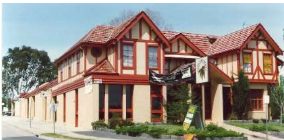
Eltham Hotel (pre 1940 section), 746 Main Road, Eltham (HO116). (Source: VHD)
