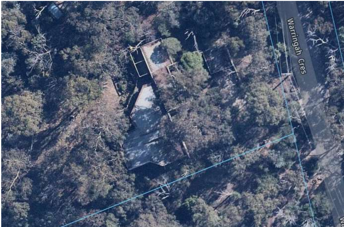
Figure 8. Aerial view showing the two sections of the house with a front single storey block of interconnecting rectilinear volumes and the rear spaces orientated towards the north (Source: Nearmap 2021)
