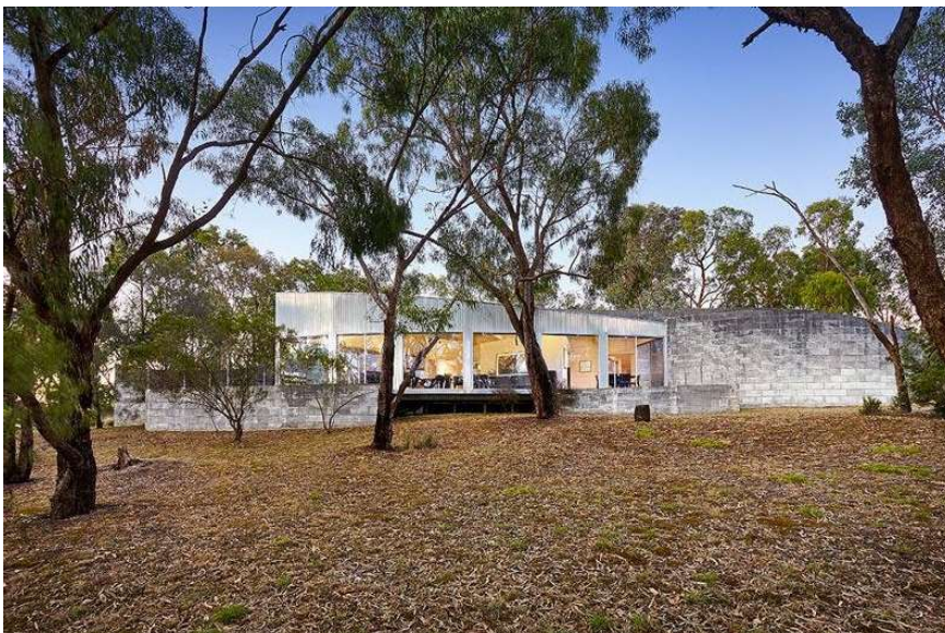
Figure 2. Southwestern elevation of the Choong House, 10 Diosma Road, Eltham. (Source: realestate.com.au 2016)
