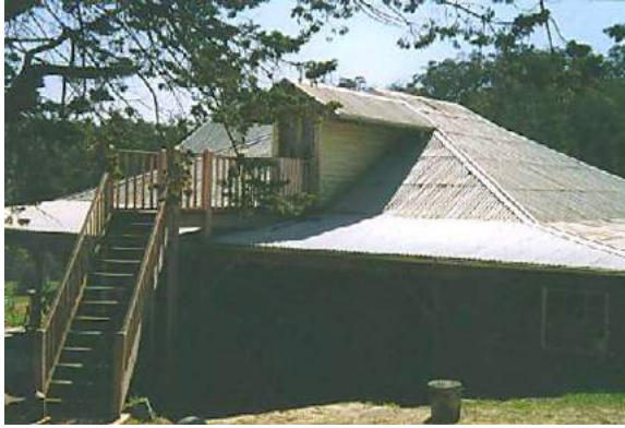
Shaw's Cool Store, 345 Hilderbrand Road, Cottles Bridge (HO212). (Source: HERMES no 66286)
