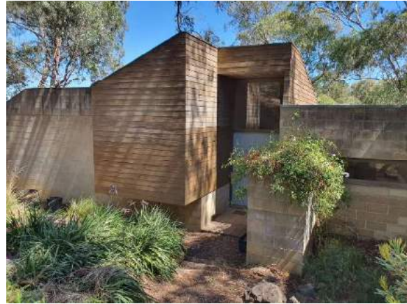
Figure 5. Entry to the house is demarcated by walls clad in horizontal timber weatherboards. The entry is double height with a skillion roof (Source: Context 2021)
