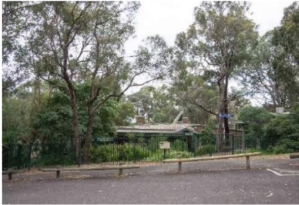
Figure 10. View of the building from the carpark. (Source: Context 2020)
