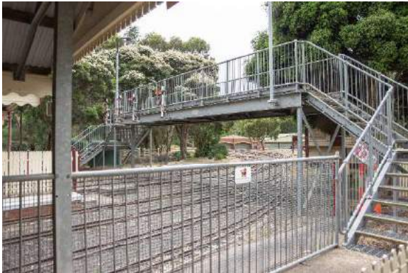
Figure 17. Steel-framed pedestrian bridge. (Source: Context 2020)
