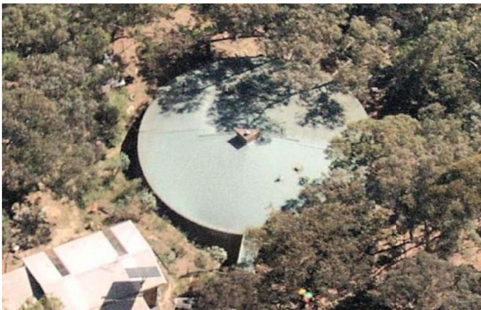
Figure 2. 57 Thompson Crescent, Research. (Source: Nearmap, November 2020)
