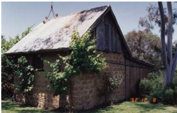
Peter Garner mudbrick studio and adjacent shed 62 Brougham street, Eltham (HO17). (Source: VHD)
