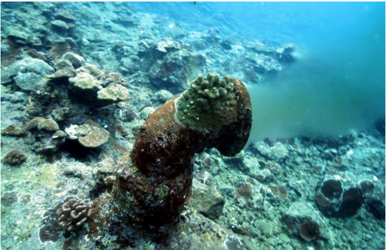
FIGURE 12. Underwater photos of East Honolulu Wastewater Treatment Plant ocean outfall off Sandy Beach, Oahu (top), and Hilo Wastewater Treatment Plant ocean outfall in Puhi Bay, Island of Hawaii (bottom). Treated sewage effluent, with high concentrations of dissolved nutrients, can be seen discharging from diffusers. Both diffuser structures are colonized by healthy reef corals of a variety of species. No benthic algal blooms or high levels of plankton that would be apparent by green water are visible. Both outfalls have been in operation for decades with no impacts to surrounding biota.
