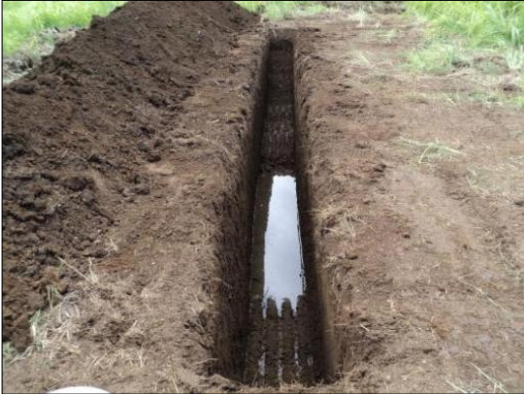
Figure 89. ST-4 view to east.
