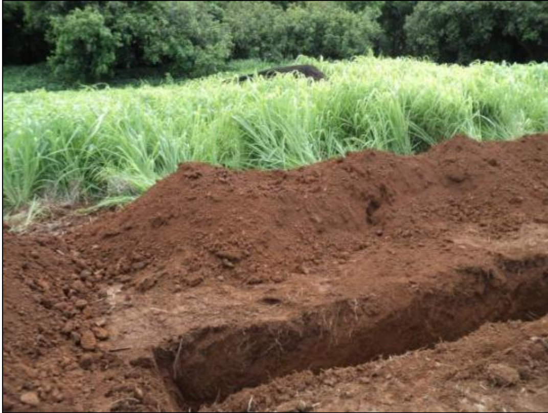
Figure 100. ST-11 view to north.
