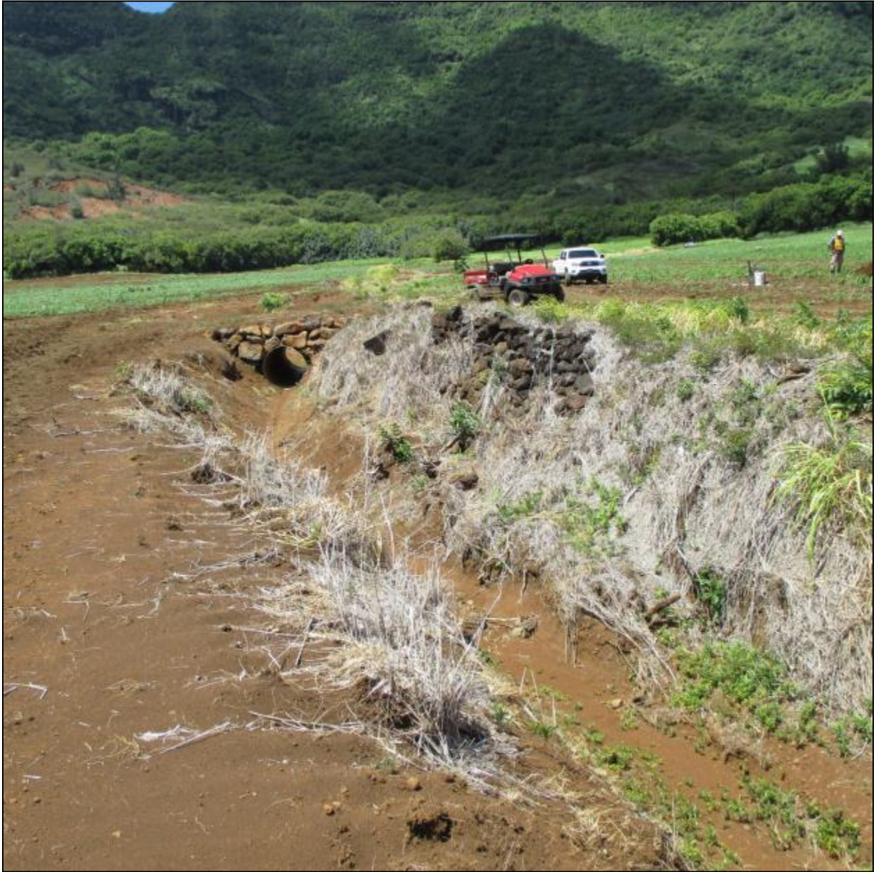
Figure 38. Site -2254 retaining wall and Site -2255, Feature 1 (culvert). View to north.
