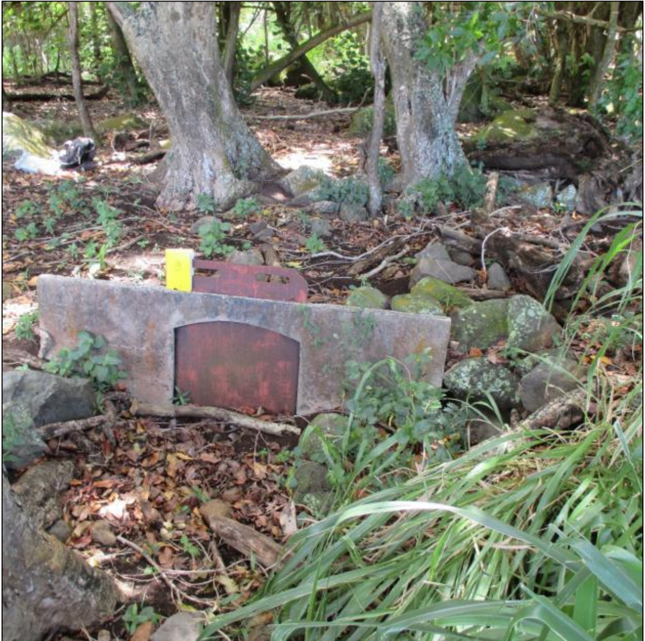
Figure 32. Site -2252, Feature 2 sluice gate. View to northwest.
