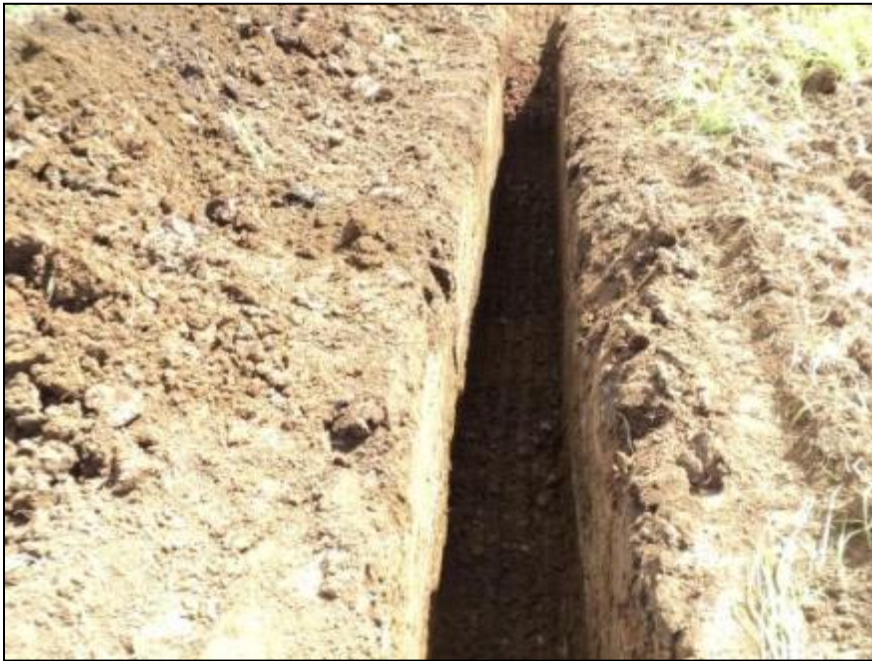
Figure 106. ST-16 view to north.
