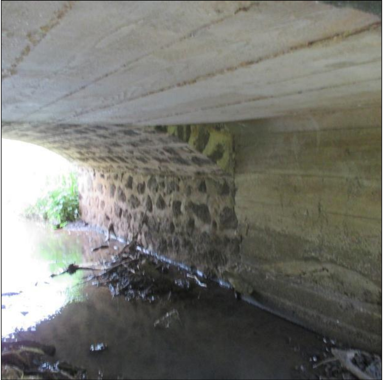
Figure 55. Site -2261 bridge, showing 1908 section and 1951 section. View to northeast.
