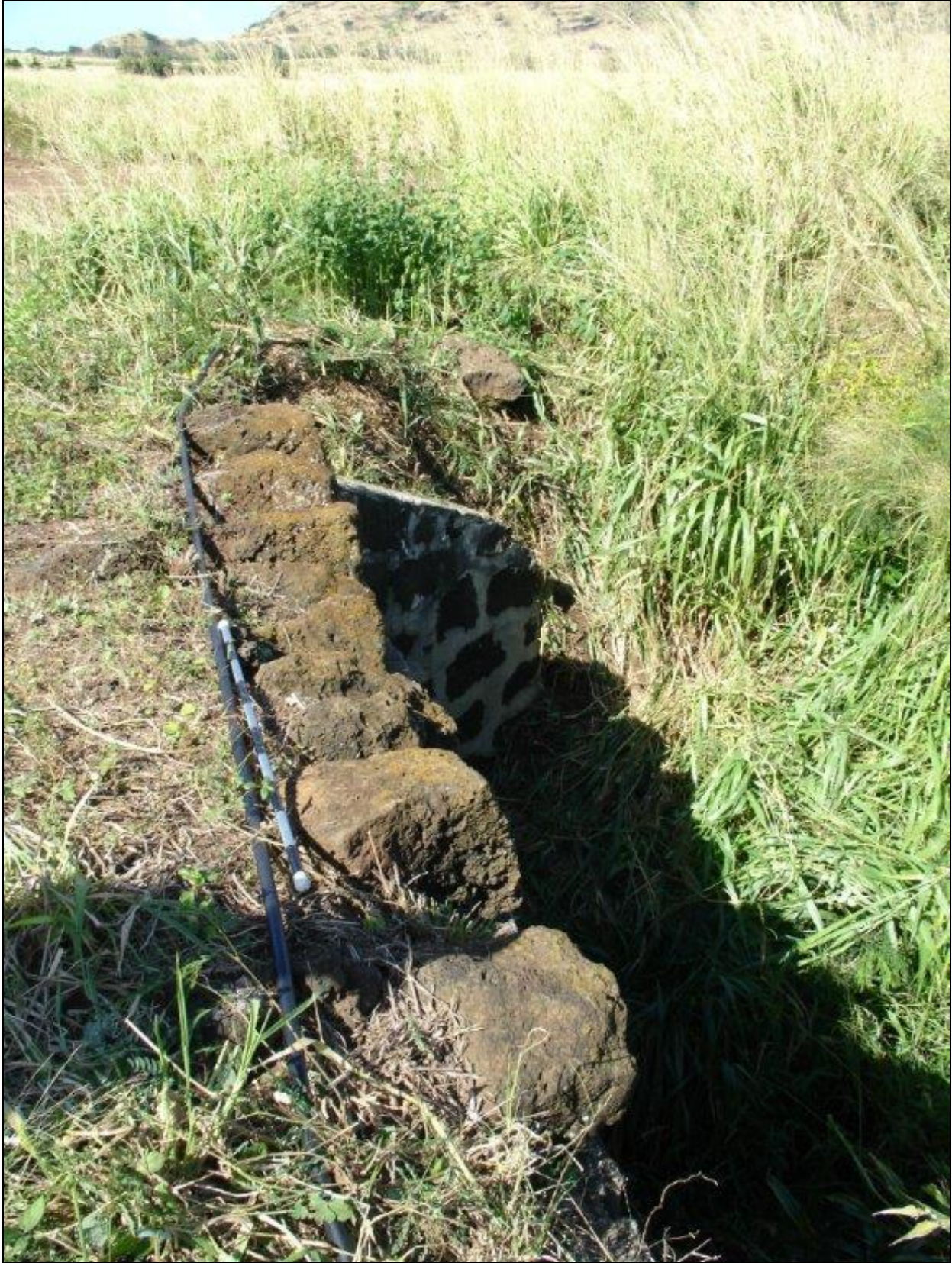
Figure 56. Site -2261, '1908' section, view of north parapet. View to north.
