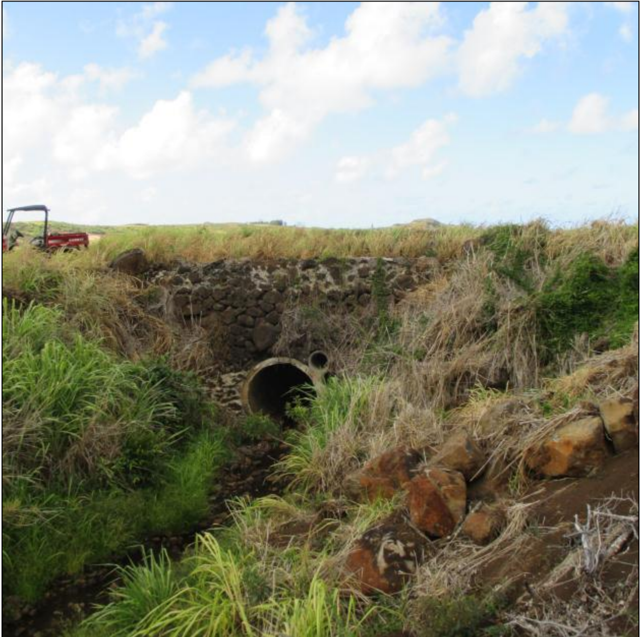
Figure 58. Site -2263 bridge. View to south.
