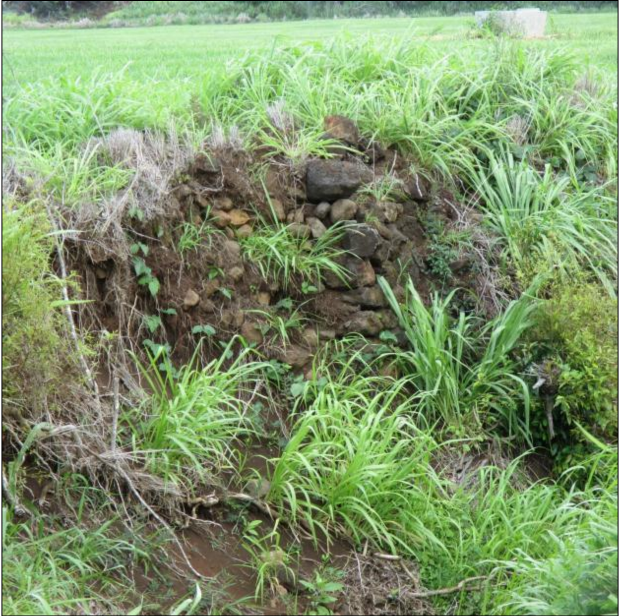
Figure 47. Site -2257 retaining wall remnant. View to southwest.
