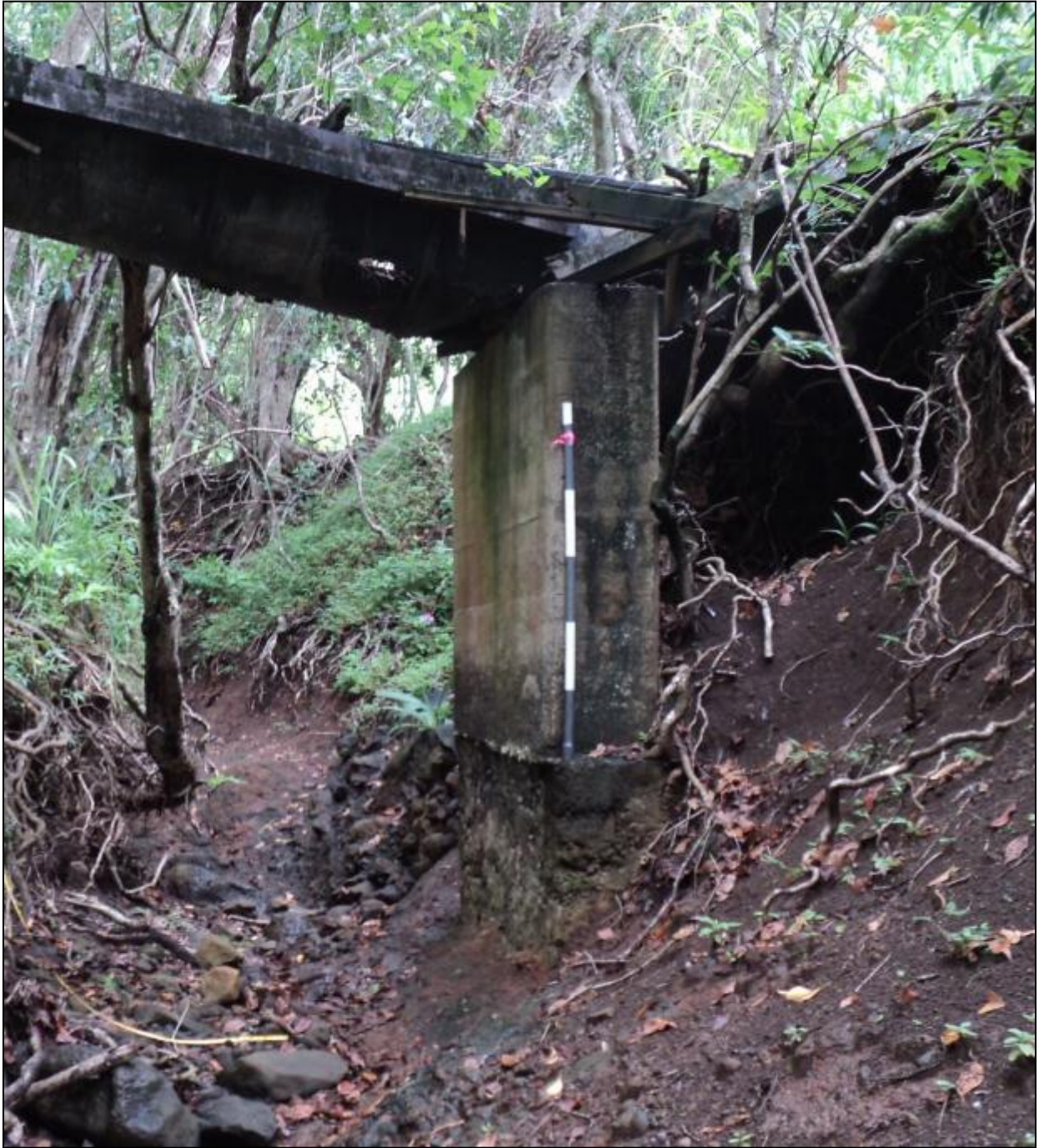
Figure 66. Site -2262 north bank foundation. View to north.
