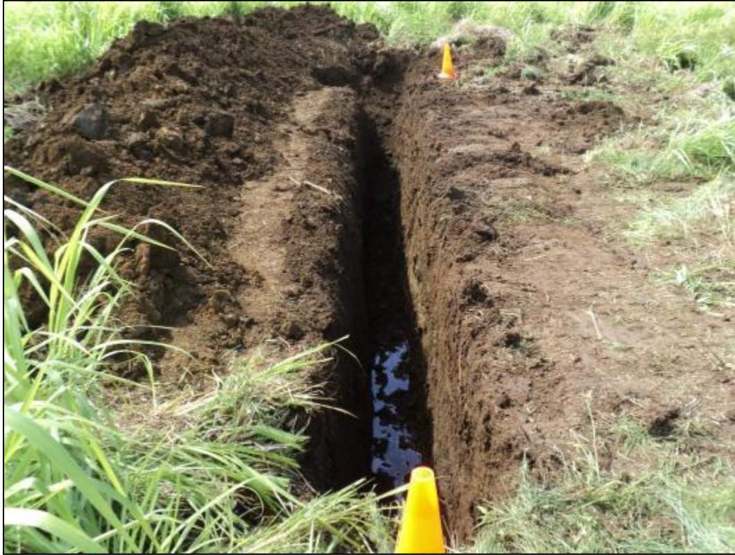
Figure 83. ST-1 view to east.
