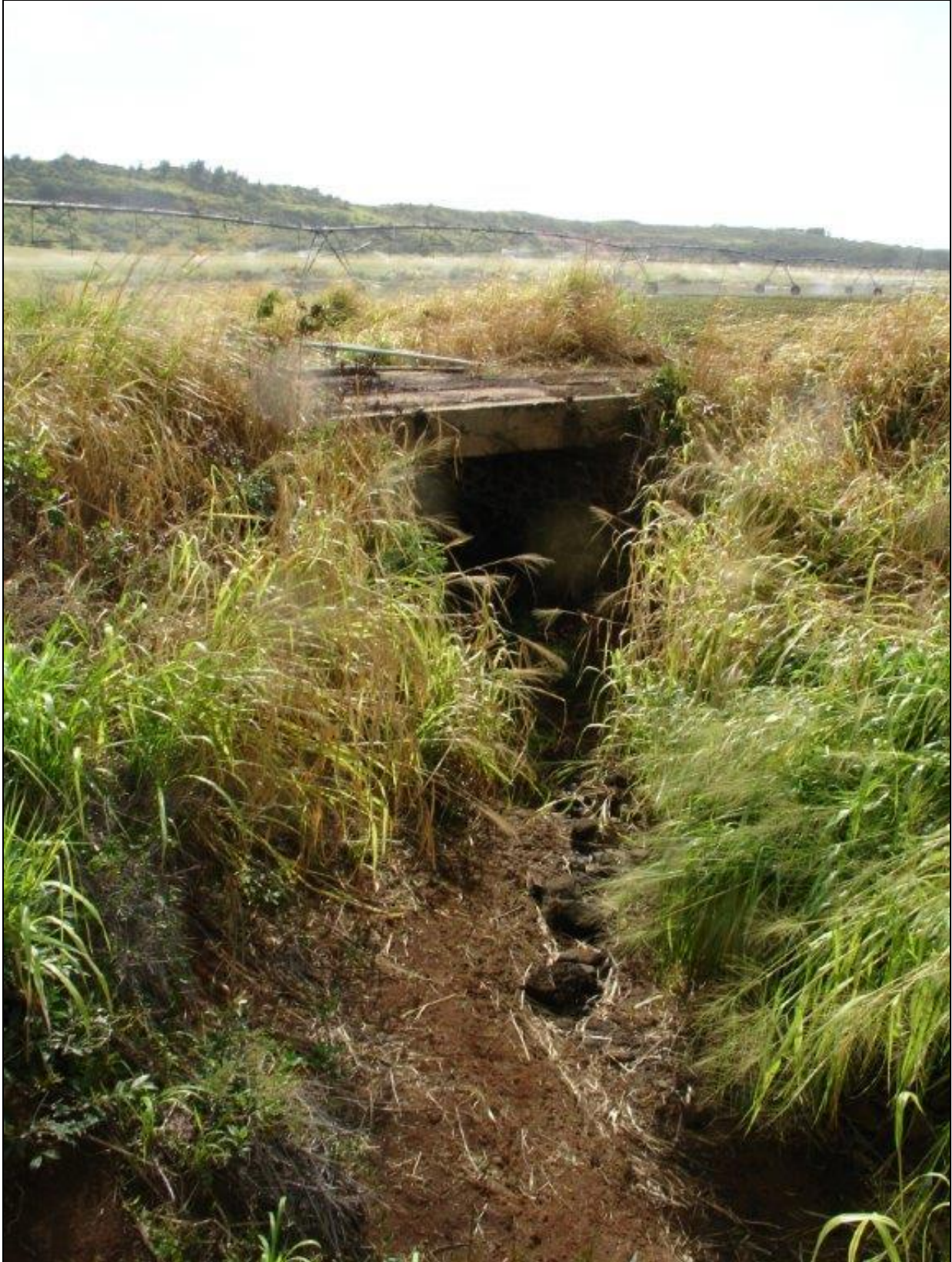
Figure 43. View to southeast of Site -2256 bridge.
