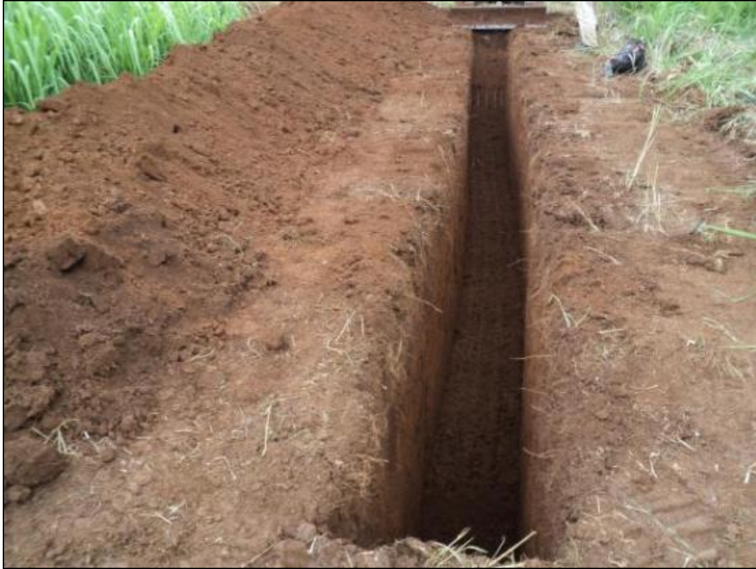
Figure 98. ST-10 view to east.
