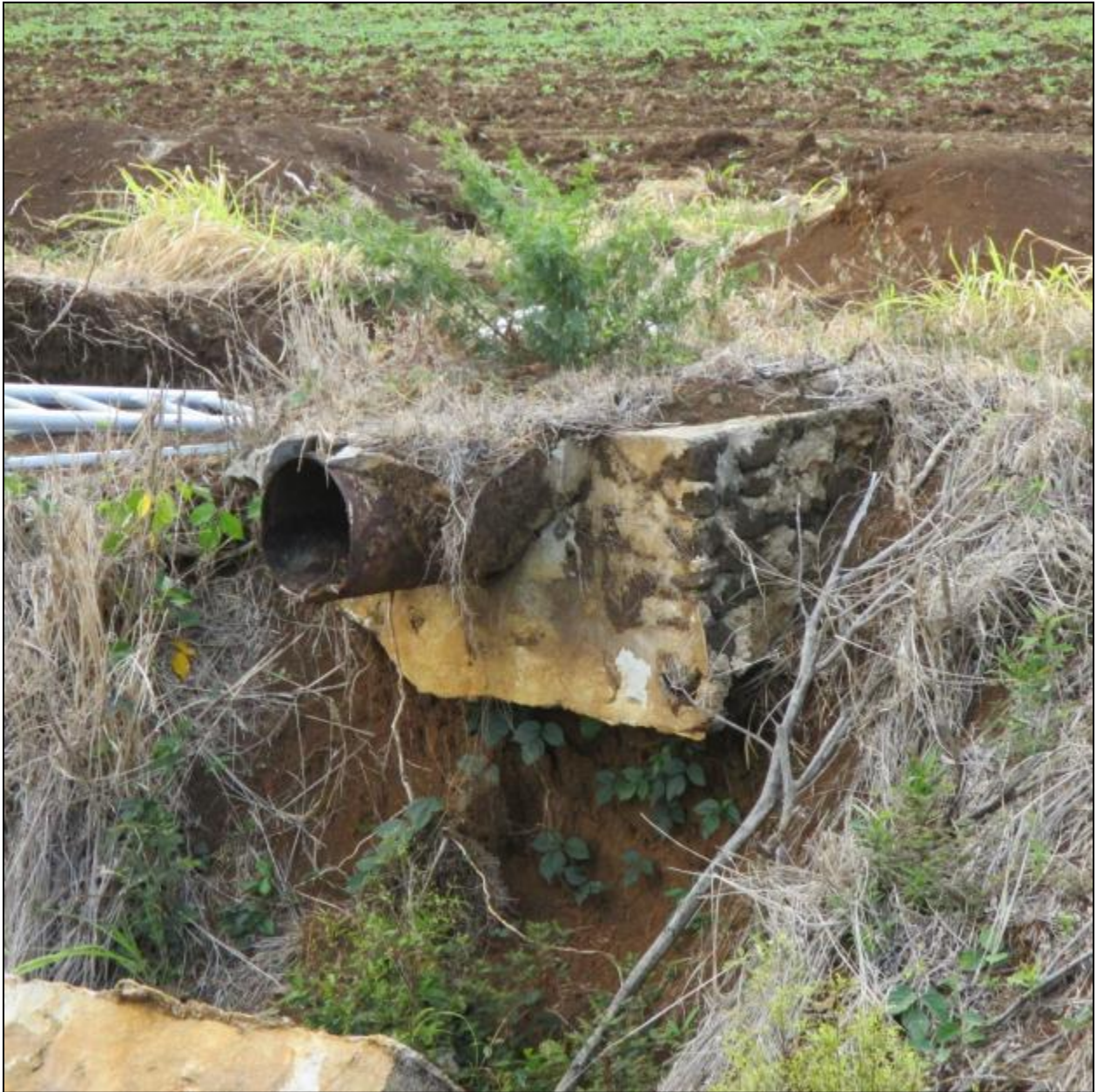
Figure 60. Site -2264 culvert and pipe. View to northeast.
