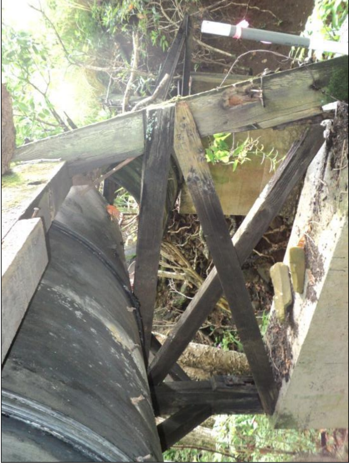
Figure 65. Site -2262 structural supports of the flume. View to east.
