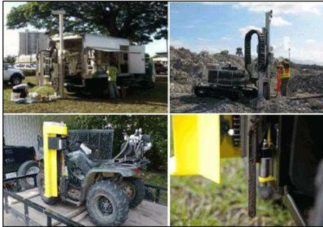
Figure G-2. Direct push drill rigs.
