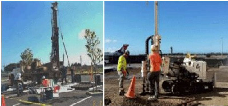
Figure G-11. Hollow-stem auger drill rig.
