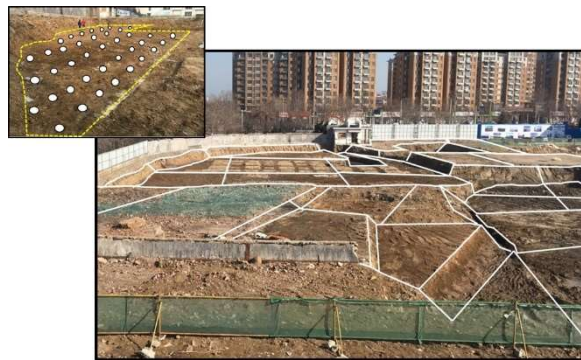
Figure C-24. Designation of excavation floor and sidewall DUs for the collection of Multi Increment confirmation samples after initial soil removal.
