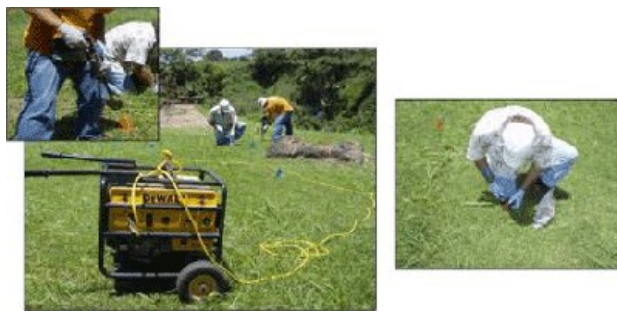
Figure F-14. Use of an Electric Hammer and Spade Bit.
