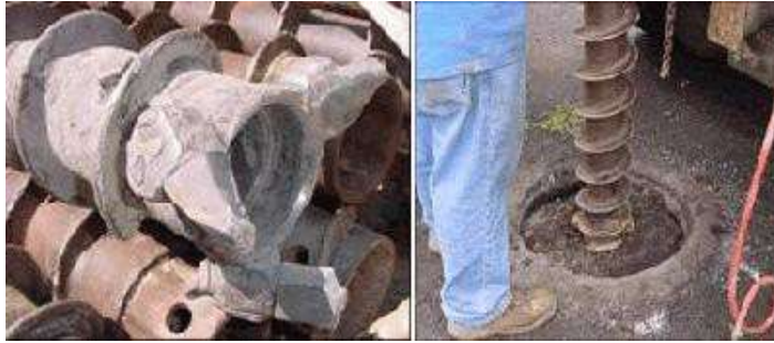
Figure G-12. Auger drill bit and drill string.
