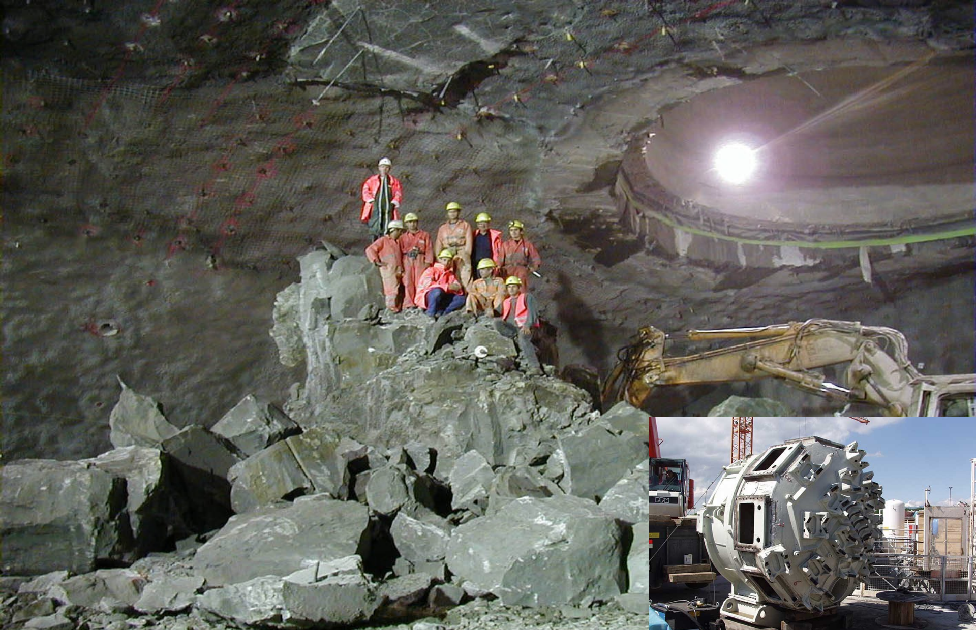
Point 1 - UX15 vault demolition of central pillar - September 20, 2000 - CE
