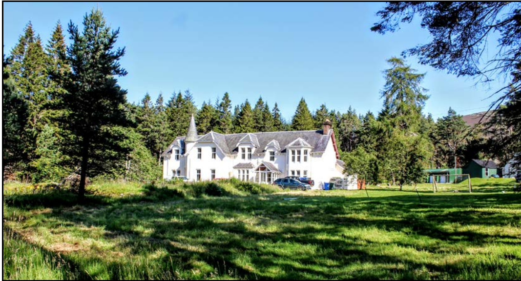
Photograph 15-2: Drumochter Lodge (Asset 7.18) looking north-east
