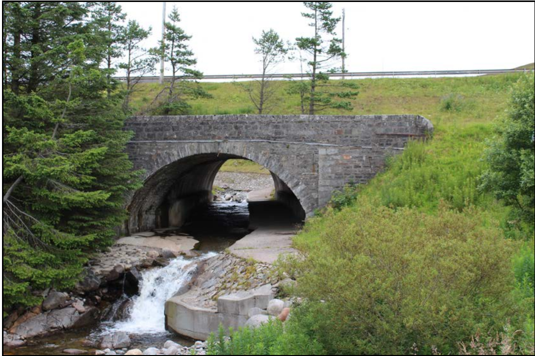
Photograph 15-3: Dalnaspidal Bridge (Asset 7.4) looking south-east
