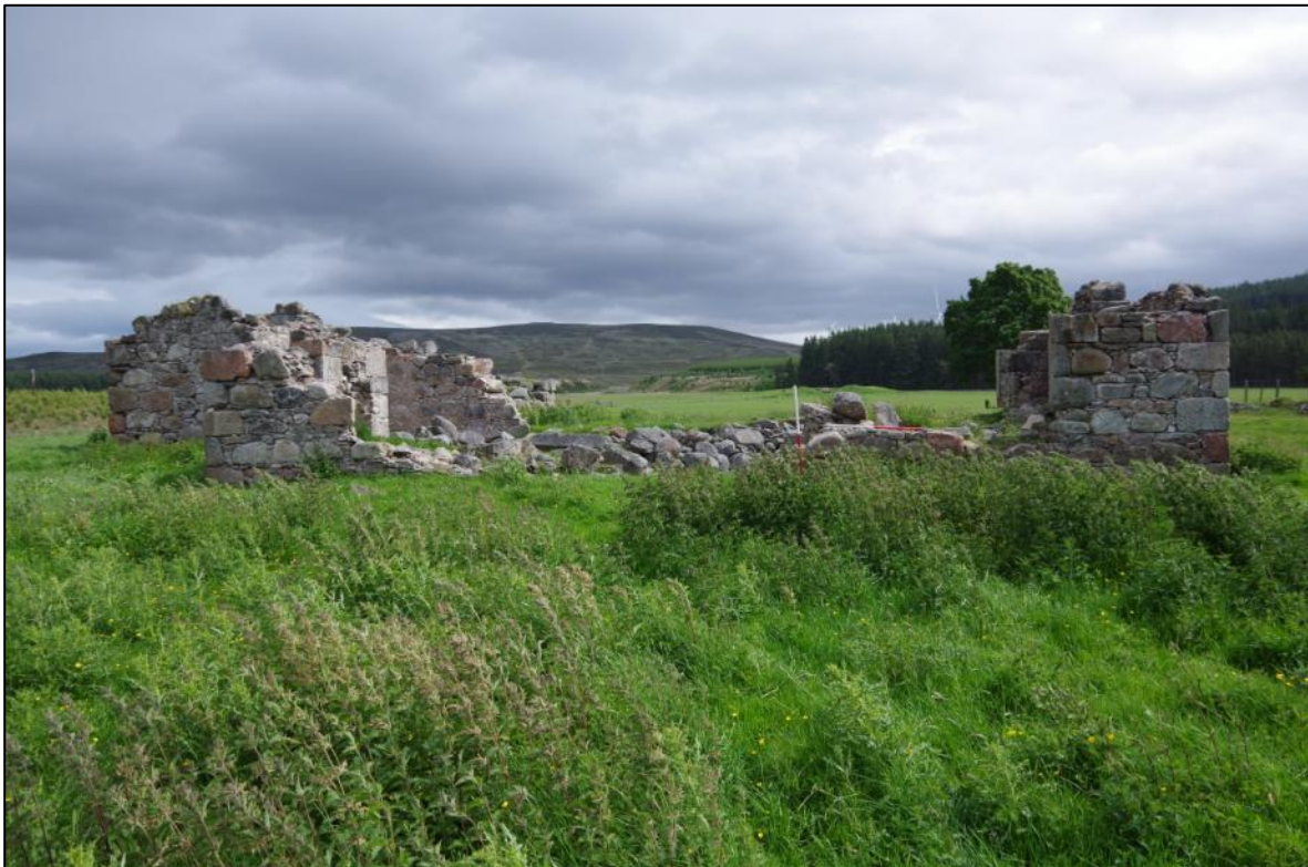
Figure 11: Photo showing W10a in center and W10b gable visible on left (1m scales, photo 7212)
