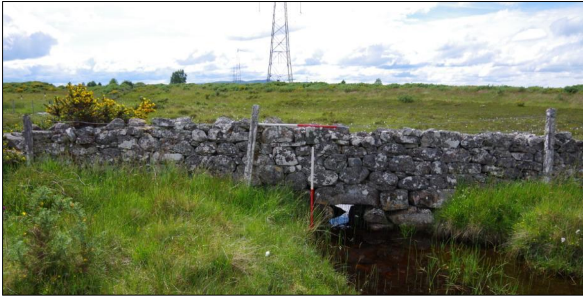
Figure 18: Photo showing W30 dry stone wall (photo 7290, 1m scales)
