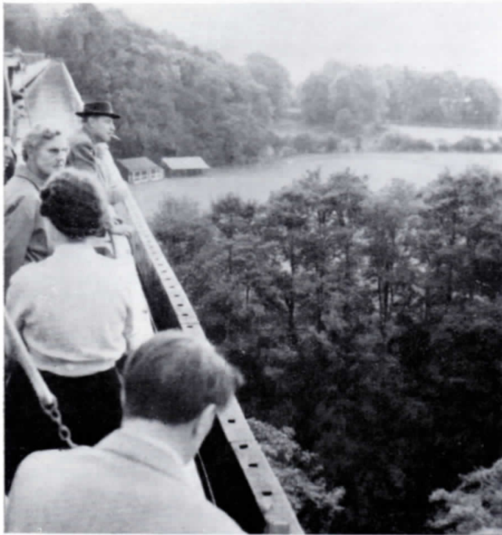
Crossing the Aqueduct
