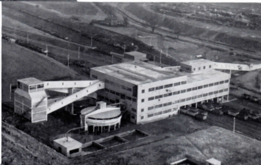
CALVERTON COLLIERY — Coal Preparation Plant, handling 450 t.p.h. Run-of-mine coal.
