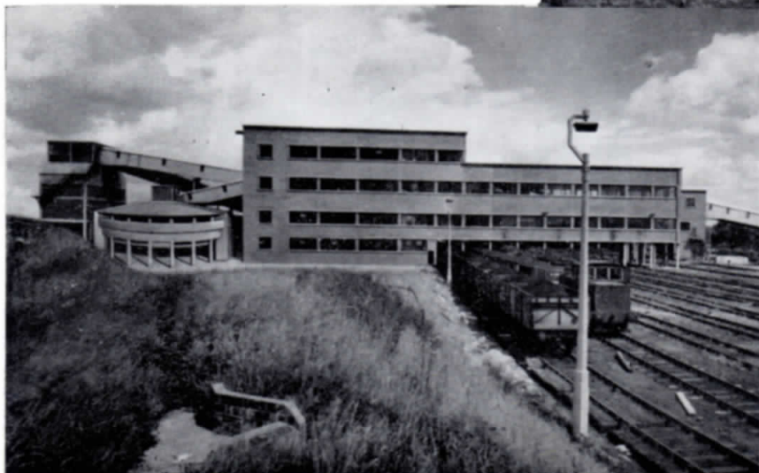
Another view of Calverton Colliery Coal Preparation Plant.
