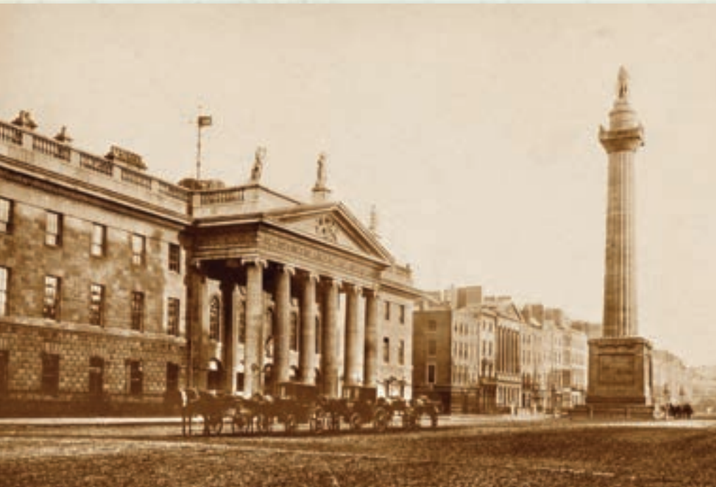
Above: A postcard (1865) showing the neo-Classical ensemble formed by the GPO and the adjacent Nelson's Pillar. As symbols of imperialism, both were ultimately targeted by nationalists seeking or commemorating independence: the GPO was occupied on Easter Monday 1916 while the pillar fell on the fiftieth anniversary of the Rising in 1966.
