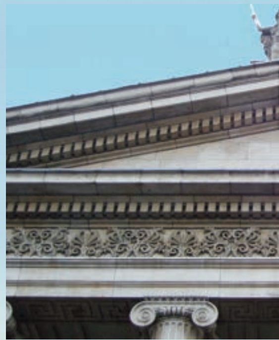
Above: Just as the royal insignia on post boxes would come to of post offices across the country, were removed or replaced. A stone work, is the only physical evidence of the long-lost coat of
