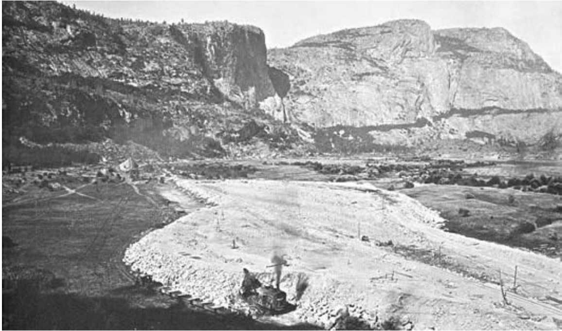
Figure 5.1: This sand and gravel operation in Hetch Hetchy Valley provided material for construction of O’Shaughnessy dam. (Photo credit Tuolumne County)
