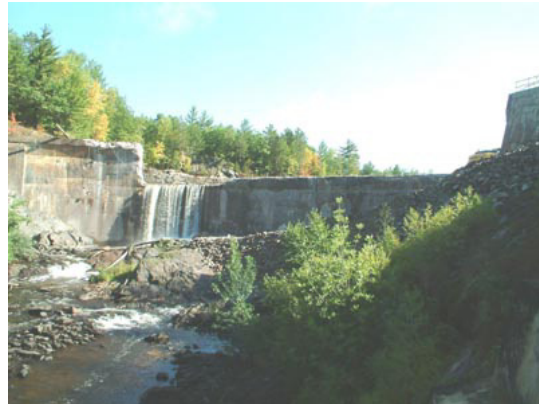
Figure 4.1: Sturgeon River Dam after phase one of deconstruction (Michigan 2004).
