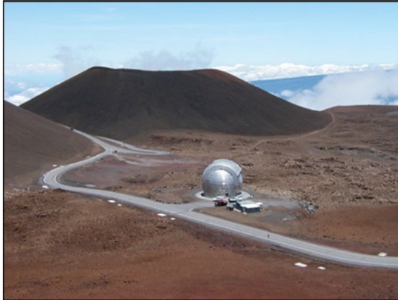
The CSO stands beside the Mauna Kea Access Road. Source: Caltech (2019)
