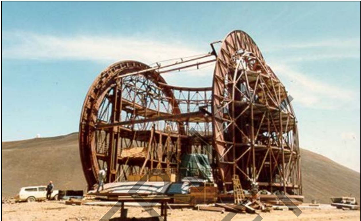
Figure 5-5: CSO's Internal Structure During Construction
