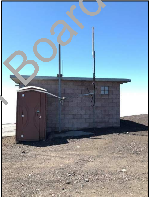
Figure 3. Top: Hōkū Ke'a Observatory, View to the South. Bottom: Hōkū Ke'a Generator Building, View to the West.
