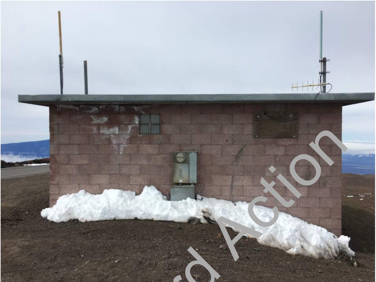
Rear view of Generator Building. (Source: PCSI)
