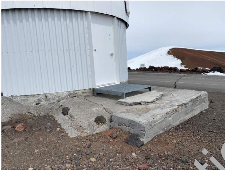
Present-day view of original door location in Observatory. (Source: PCSI)
