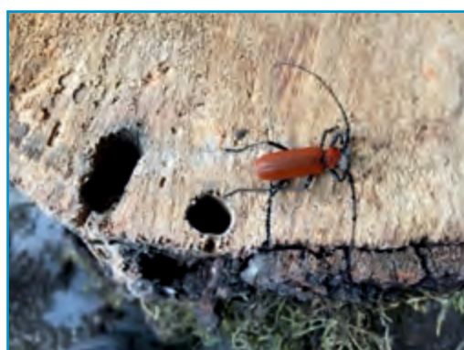
(c) Exit holes on kharsu oak logs
