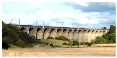
each spanning 15.2m (50 feet), together with 3 at the east end, each of span 6m, leading from an embankment. The 4<sup>th</sup> and 5<sup>th</sup> arches from the east end cross the river, at a height of 24.6m above the mean water level.
