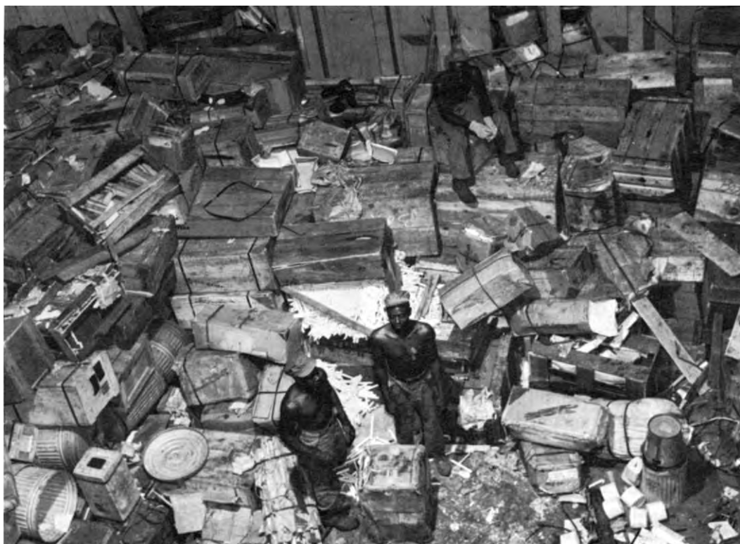
DAMAGE TO SUPPLIES caused by improper packing, dunnage, and handling.
