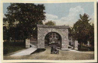
Built in the days of horse and buggy, the arch proved too narrow for modern traffic.
