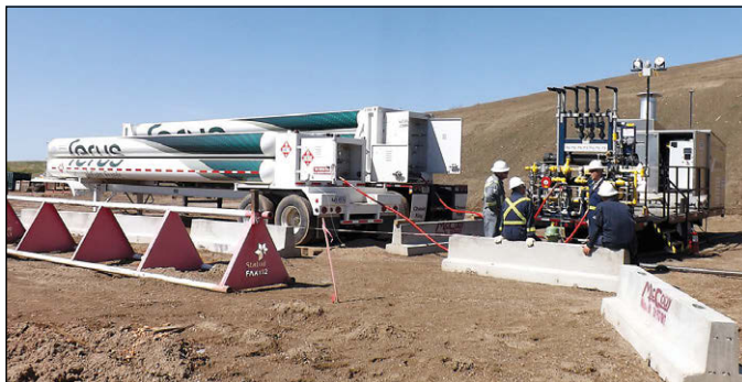
CNG is transported in Ferus tube trailers to a Statoil well location, then used to fuel the Sidewinder #104 drilling rig, where between 40% and 50% of the diesel fuel is substituted with natural gas. (Photo by Denis Smith).
