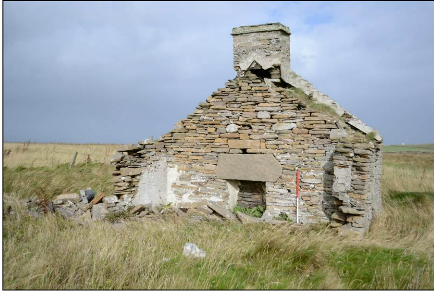
Plate 3. Later fireplace inserted into the gable end of SWC50, looking north-east.
