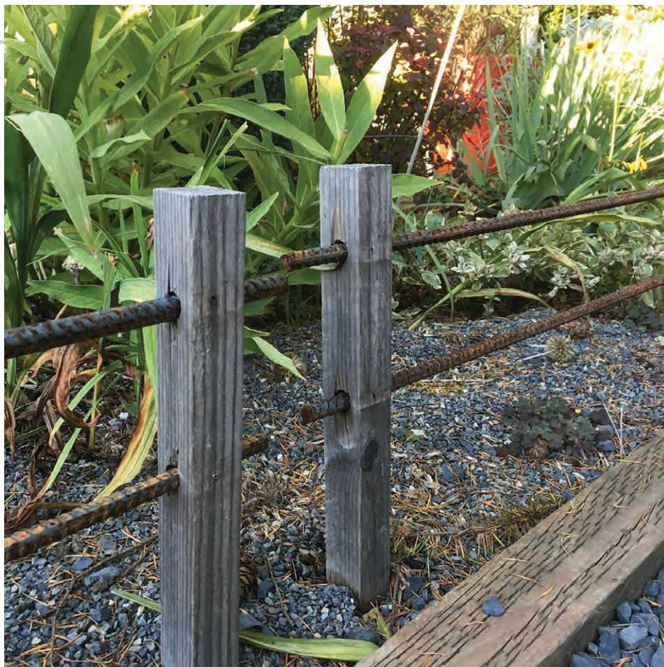
Rebar and cedar will weather to blend with most garden landscapes; pressure-treated fir posts will retain a slight orange hue.
