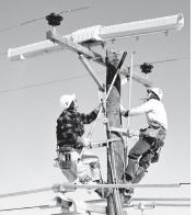
Two conductor covers lock with insulator cover on middle conductor of 34.5kV sub-transmission lines.
