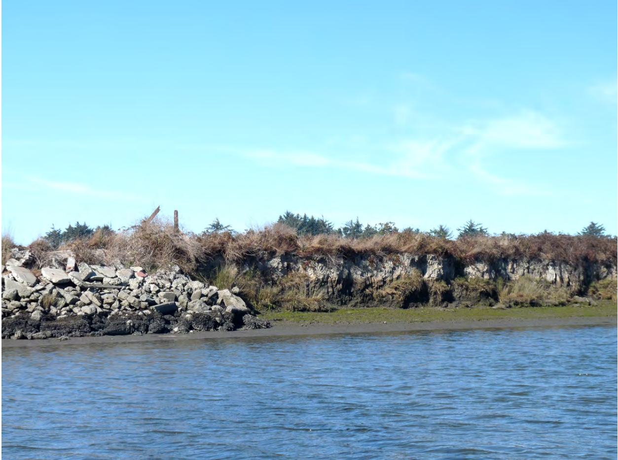
Figure 25. Mad River Slough is an example of contrasting shorelines one that is exposed and the other with concrete revetment on Humboldt Bay.
