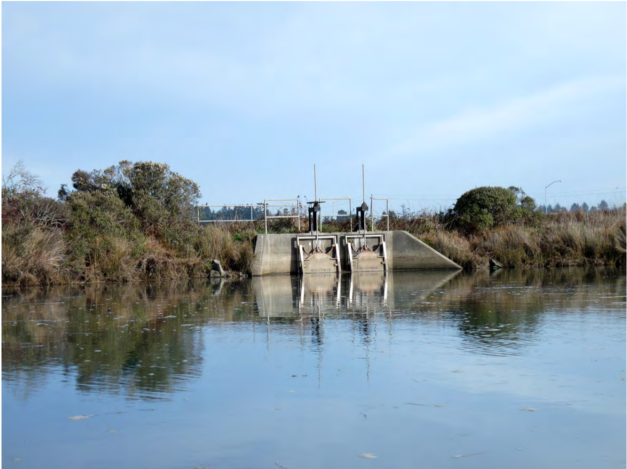
Figure 19. Elk River Slough is an example of a tidegate forming the shoreline of Humboldt Bay.
