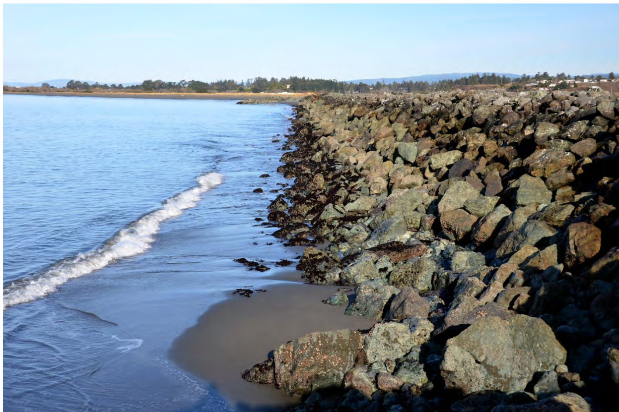
Figure 26. Eureka Bay is an example of a shoreline with rock revetment on Humboldt Bay.
