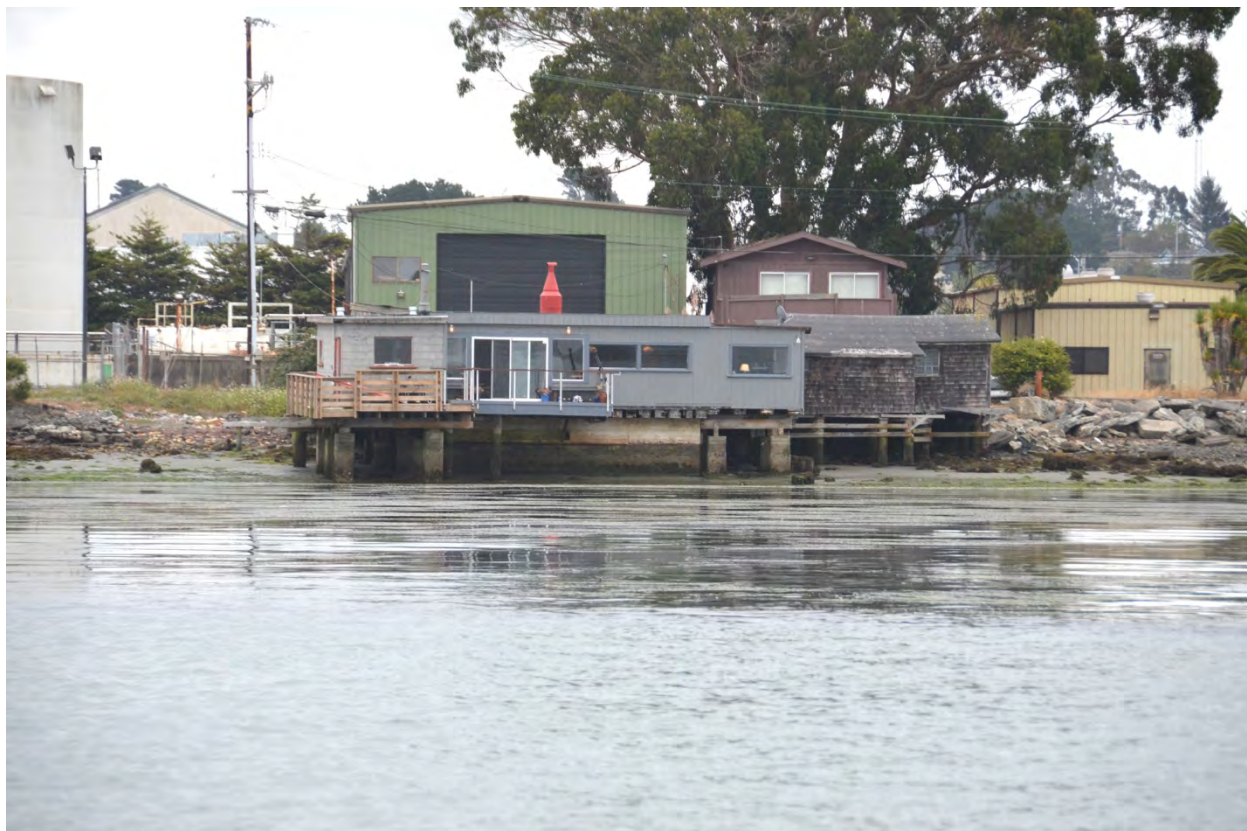
Figure 15. Eureka Bay is an example of a building and its foundation forming the shoreline of Humboldt Bay.
