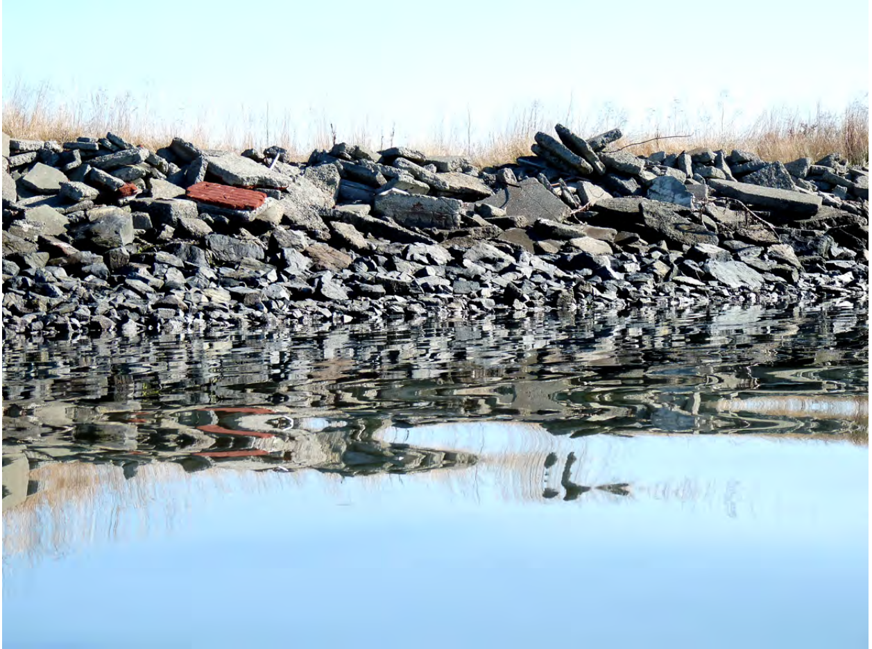
Figure 30. Arcata Bay is an example of a shoreline that is covered by a rock and concrete revetment on Humboldt Bay.
