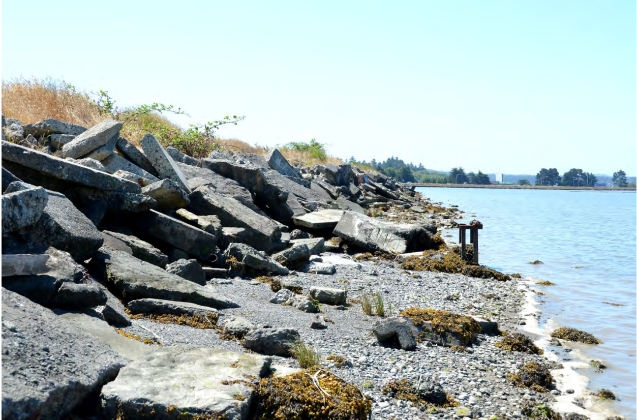
Figure 27. Arcata Bay is an example of a shoreline that is covered with concrete revetment on Humboldt Bay.
