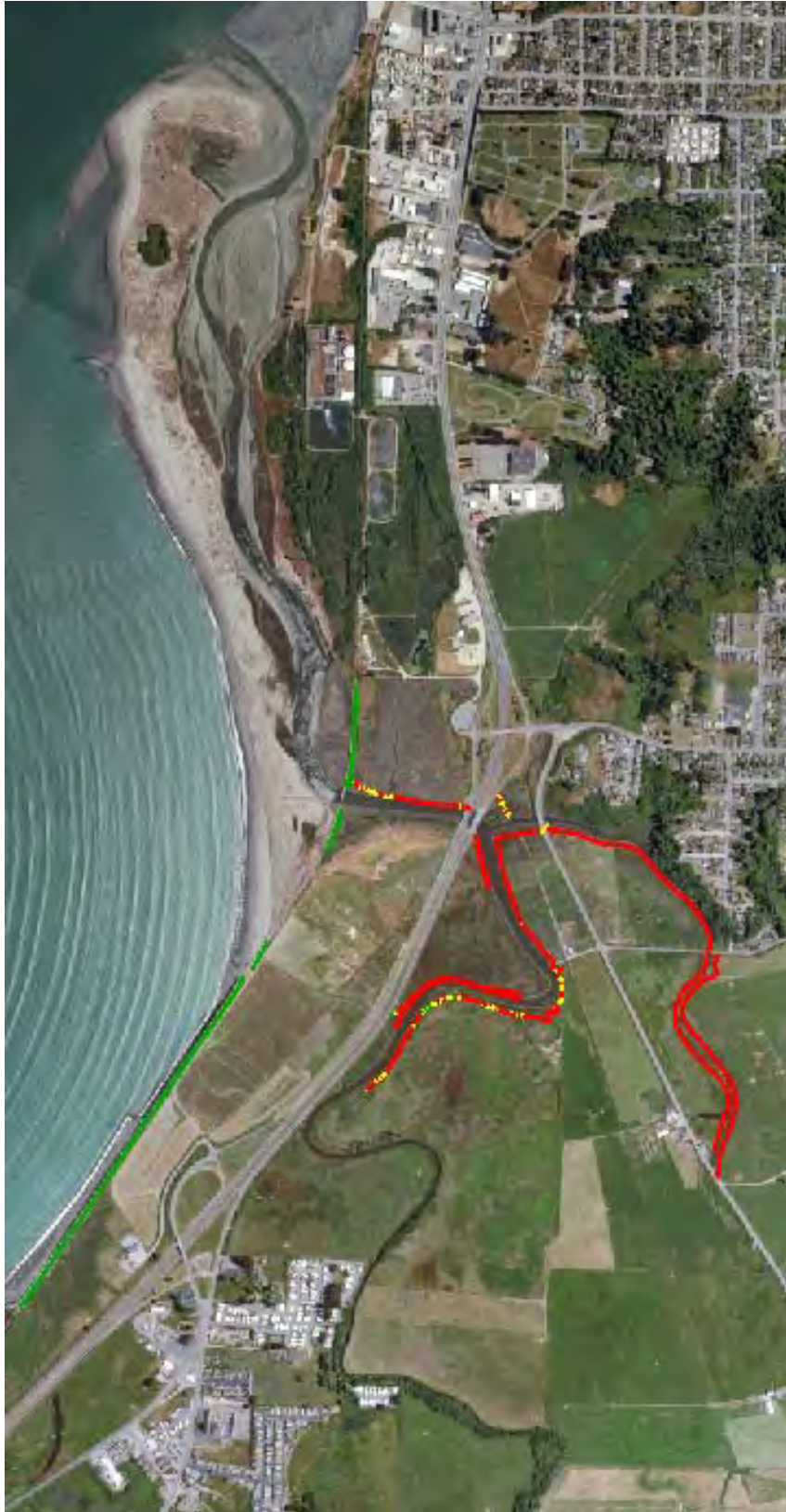
Figure 9. Diked and railroad shoreline vulnerability rating for Elk River Slough; red high, yellow moderate, and green low.
