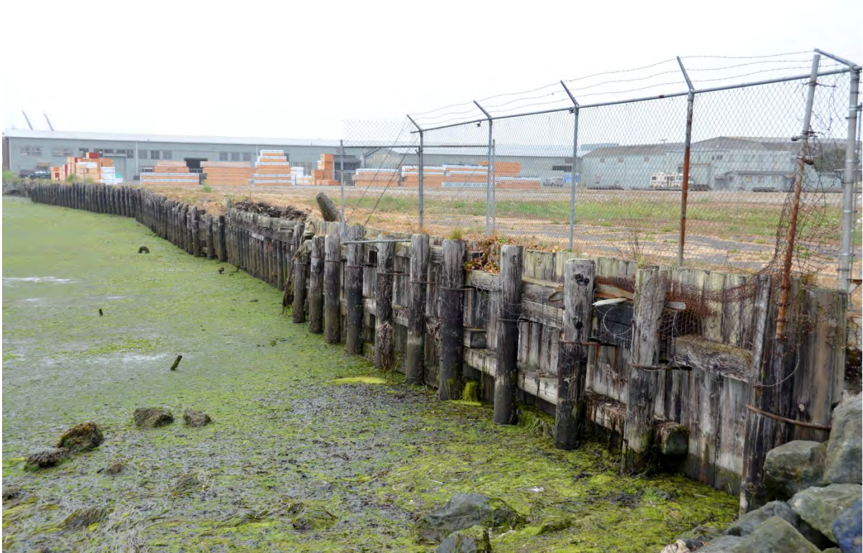
Figure 28. Eureka Bay is an example of a shoreline that is covered by a wood bulwark on Humboldt Bay.
