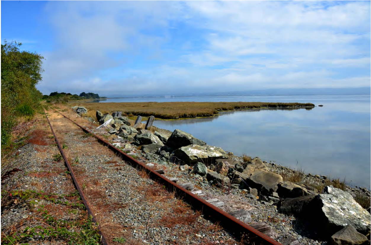
Figure 12. West-side of Arcata Bay is an example of the railroad grade on Humboldt Bay with rock revetment.
