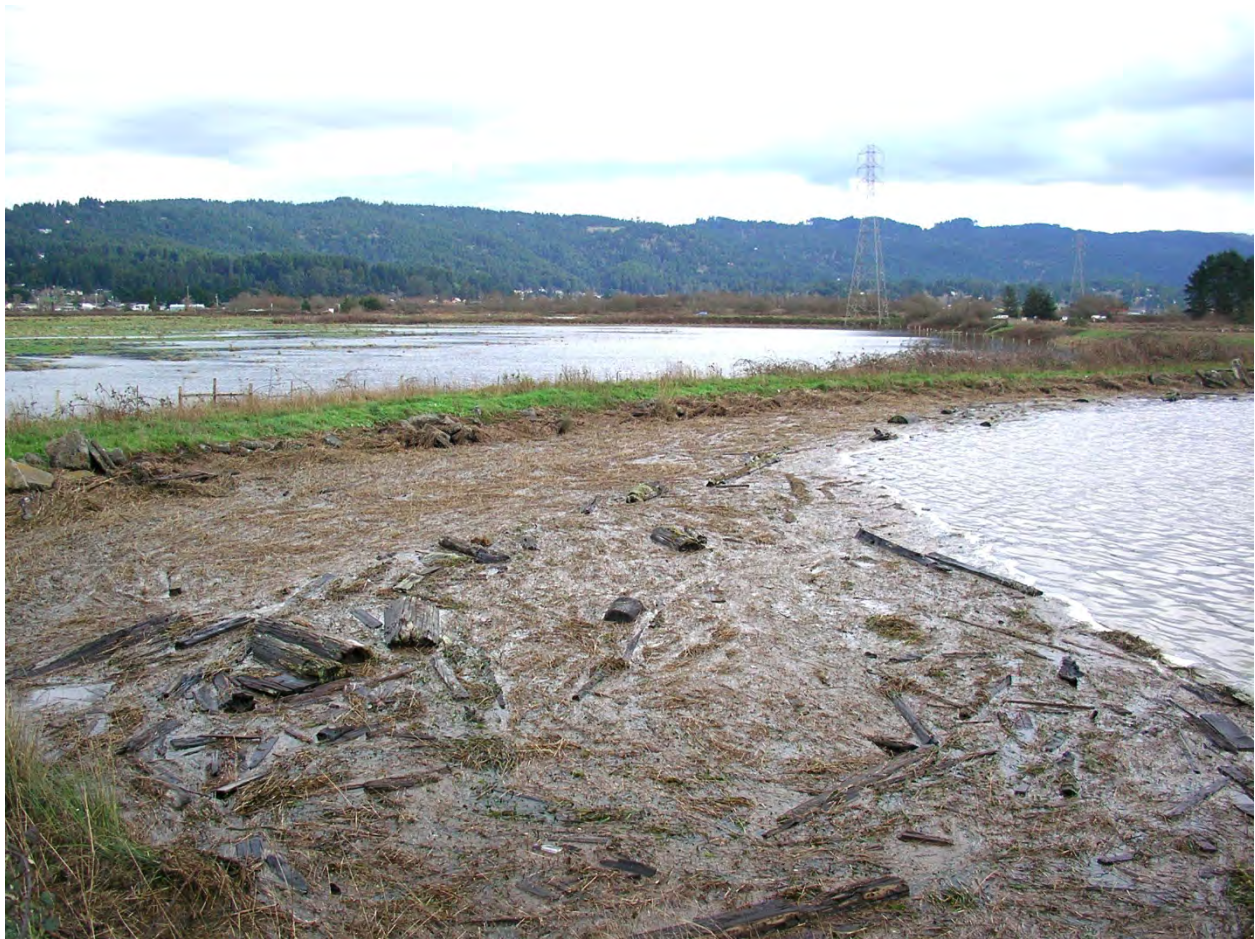
Figure 4, 2006, the maximum high tide after a period of heavy rainfall reached 9.49 feet and Arcata Bay's northern diked shoreline and City of Arcata's wastewater treatment ponds and marsh dikes were over topped in multiple locations.
