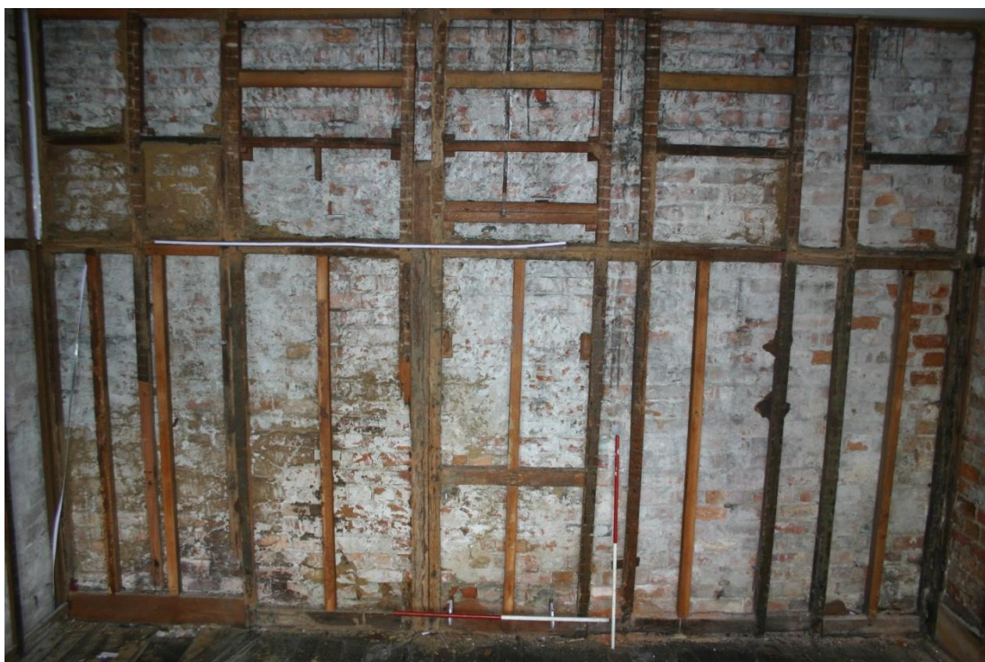
Figure 1.6 South wall in the west room. Inferred c1820s rear wall (internal) of the parsonage, with possible evidence of lathe and plaster cladding set on batons.
