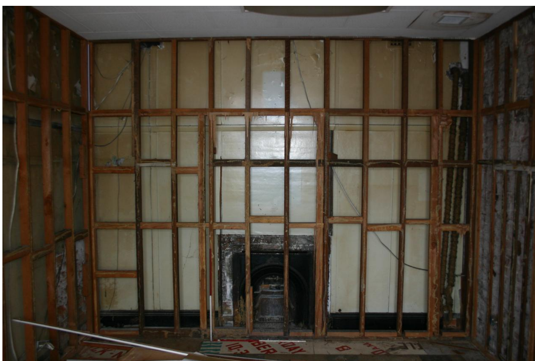
Figure 1.5 South wall in the east room of the 1902 Reception House building.
