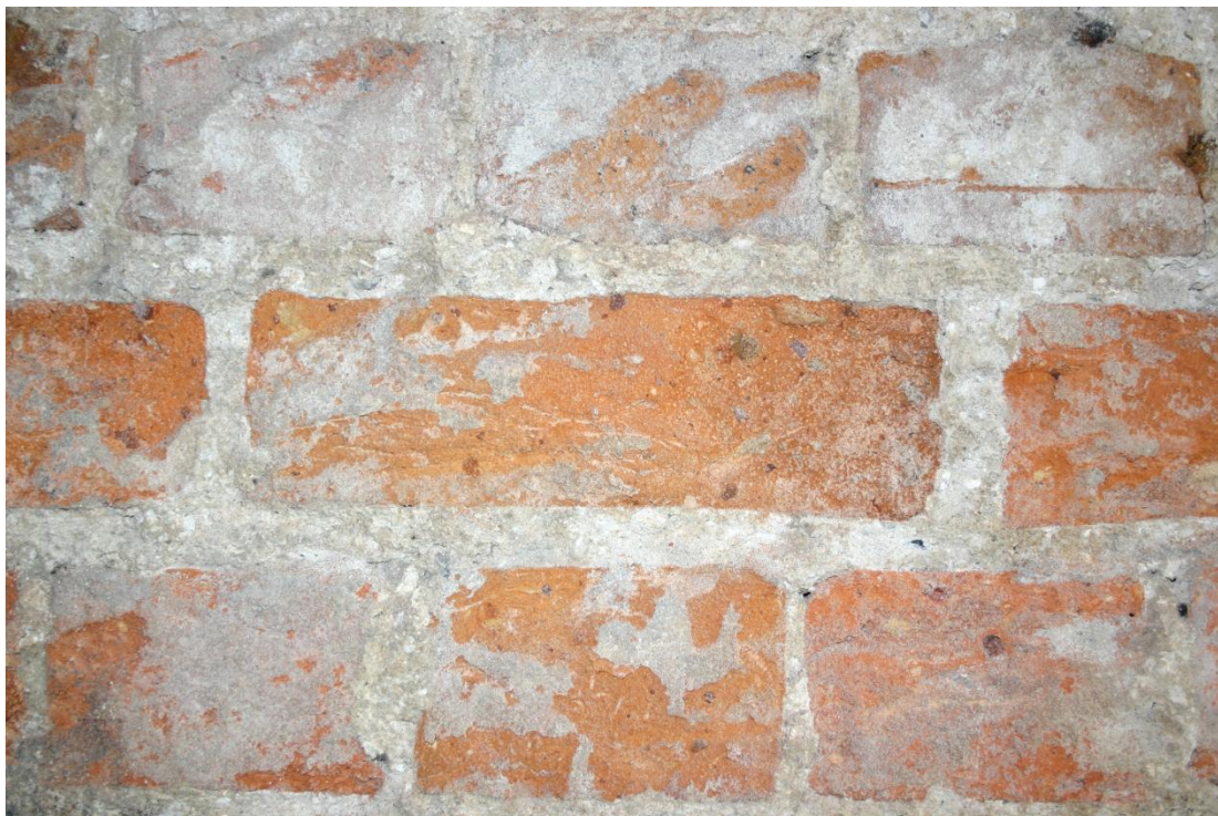
Figure.1.2 Samel-style brick (67x214mm), with fine shell lime mortar bonding. West room.
