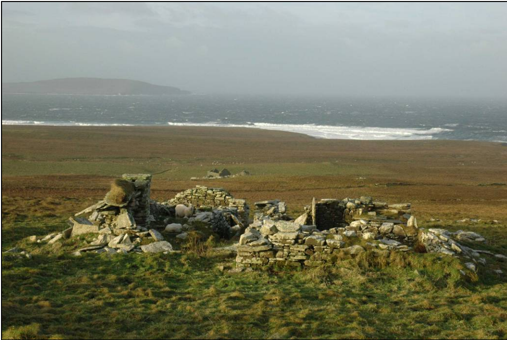
Fig. 33. The remains of Breck croft (89A)- the central place of the infield and at the heart of planning, negotiation and social stratification at the level of the household. Many features that were central to everyday routines, such as corn driers, byres, and goose nests, as well as highly personal spaces such as bed neuks and shelves survive, looking south-west.
