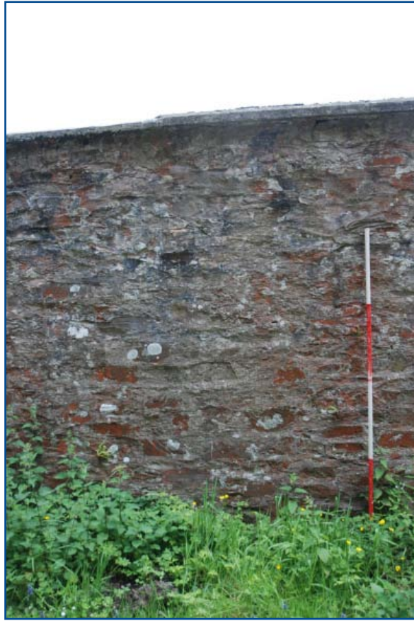
Plate 3: General view of the exterior (north-facing side) of the north wall
