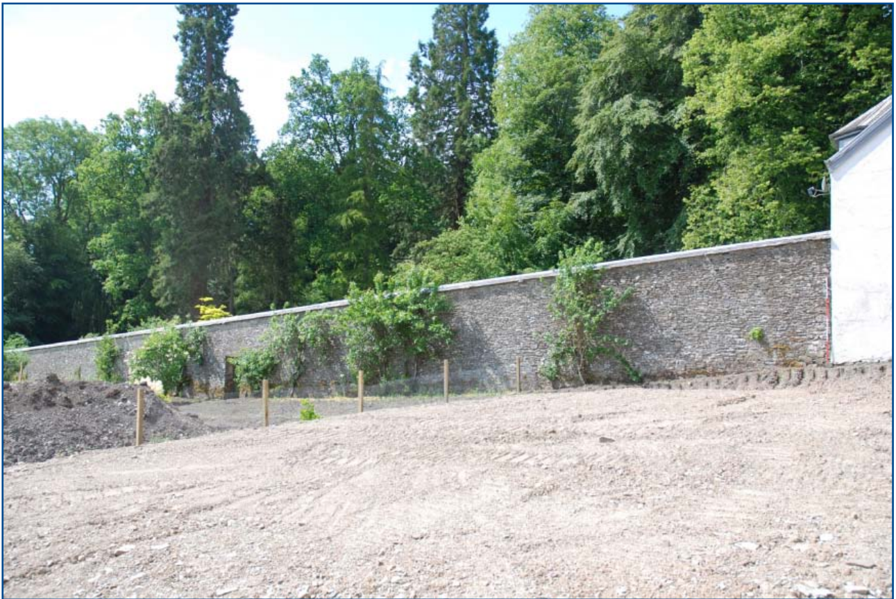
Plate 8: General view of the west wall from the NEE
