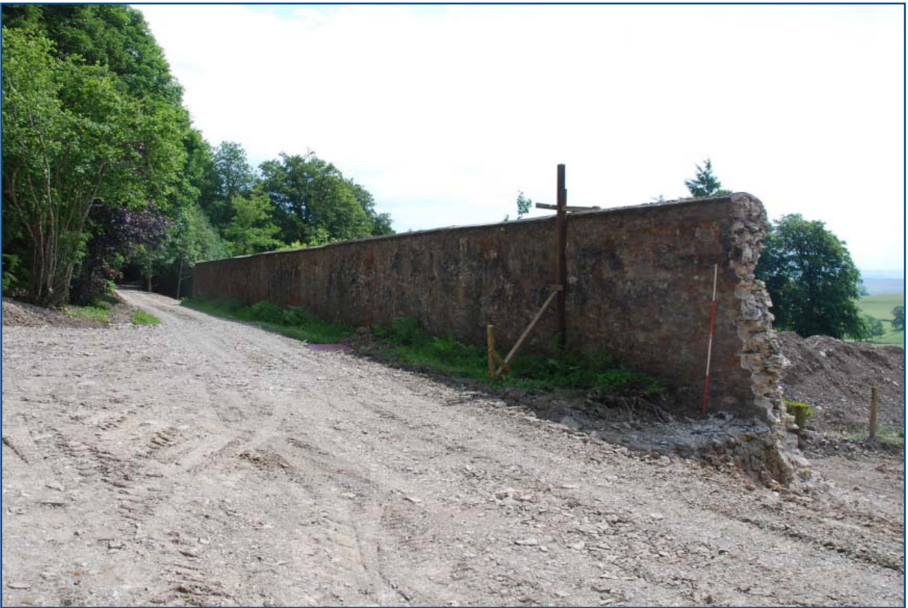
Plate 1: General view of the north wall from the north-west
