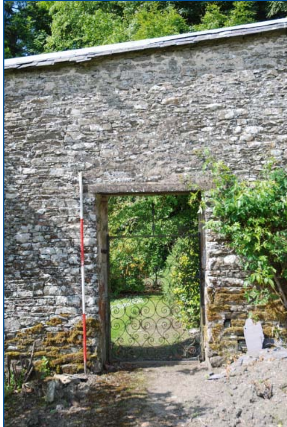
Plate 10: Detail of the doorway in the west wall from the east
