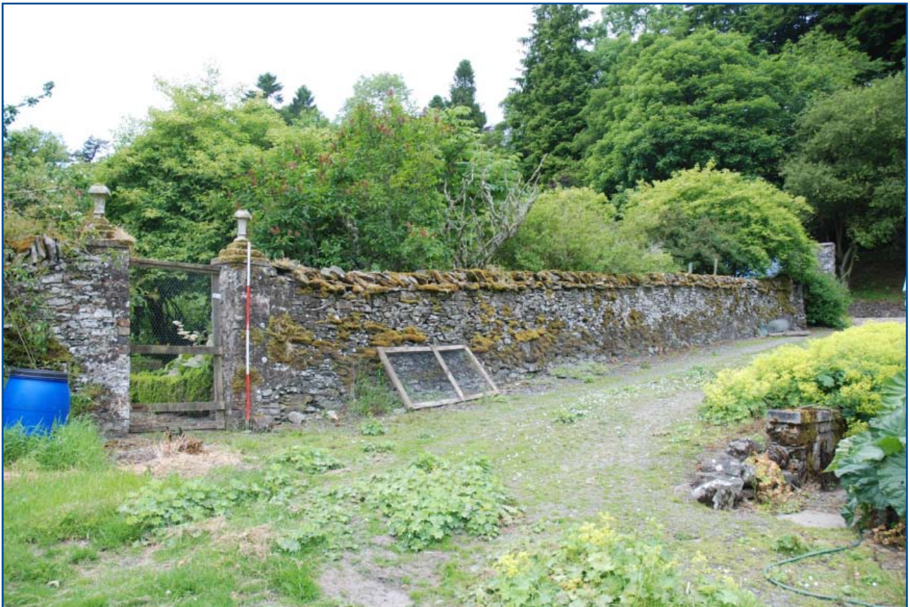
Plate 4: General view of the east wall from the south-east
