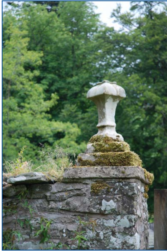
Plate 7: Detail of the finial to the doorway in the east wall
