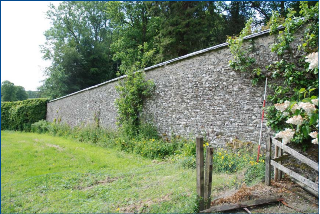
Plate 9: General view of the west wall from the north-east
