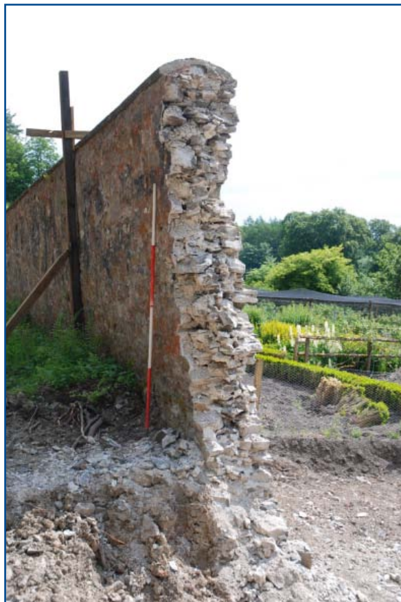
Plate 2: Detail of the demolished profile of the north wall
