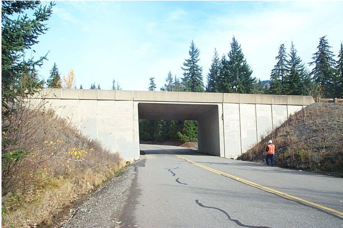
Sparks Road Bridge South. (Photo: WSDOT)
