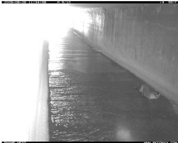
Otter in Swamp Creek West Culvert. (Photo: WTI)
