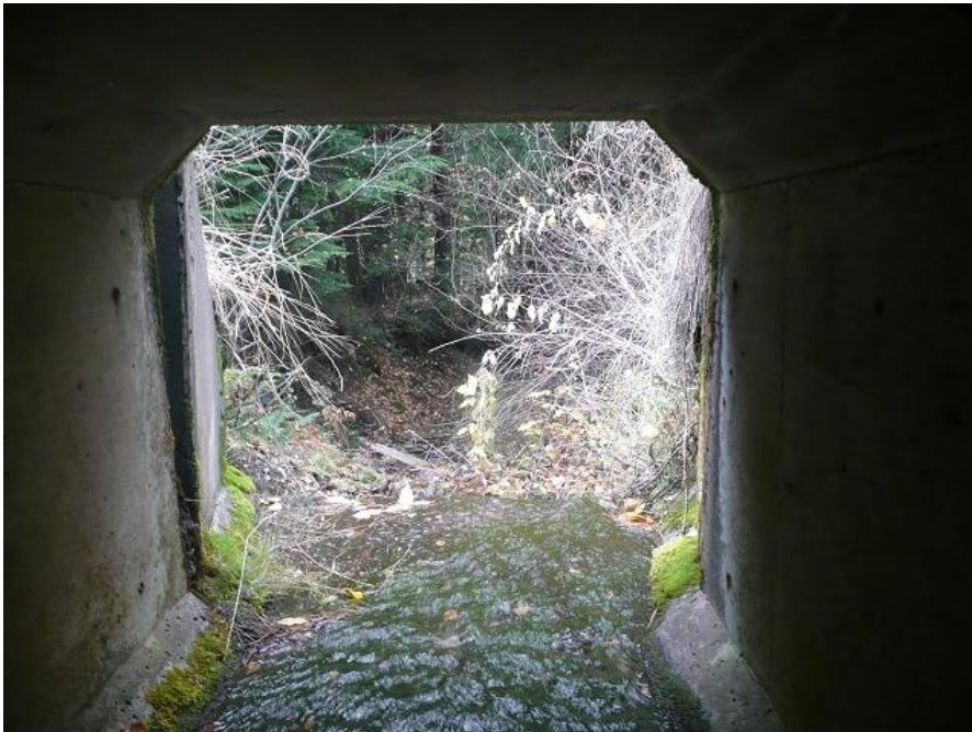
Cedar Creek Culvert north entrance. (Photo: WTI)
