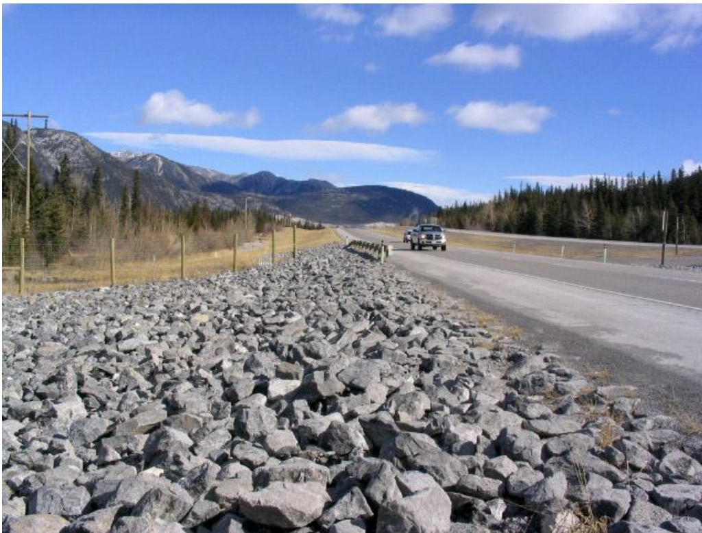
Exhibit 10. Boulder field at termination of wildlife fence on Trans-Canada Highway, near Canmore, Alberta (copyright: Tony Clevenger).
