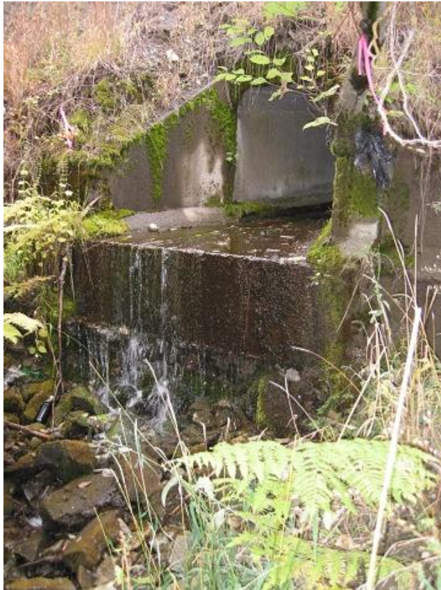
Hudson Creek Culvert south entrance with dropoff. (Photo: WTI)
