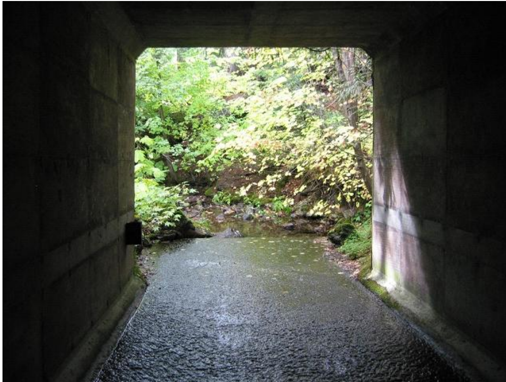
Price Creek Culvert south entrance. (Photo: WTI)
