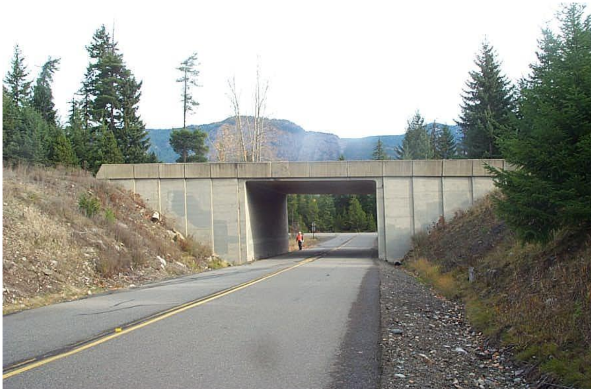
Sparks Road Bridge North. (Photo: WSDOT)
