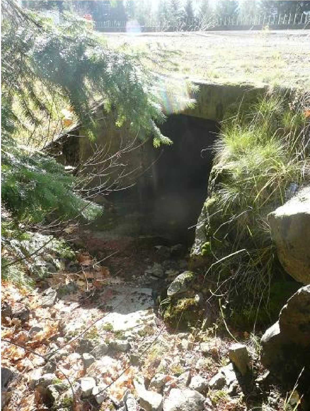
Unnamed Creek Culvert north entrance. (Photo: WTI)
