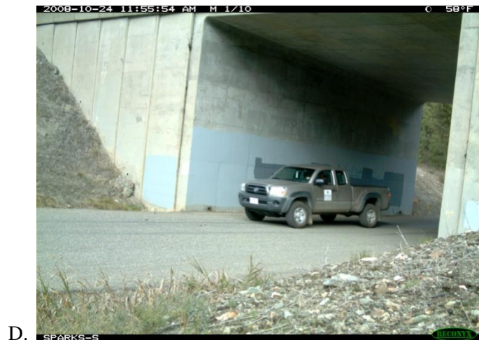
Figure 3.4. “Faux” electrical housing containing remote camera deployed at the Sparks Road Bridge South. Various images show housing (A), aim of camera (B), view from under the bridge with arrow pointing to camera box (C), and sample photo of WTI field vehicle (D). (Photos: R. Long /WTI)
