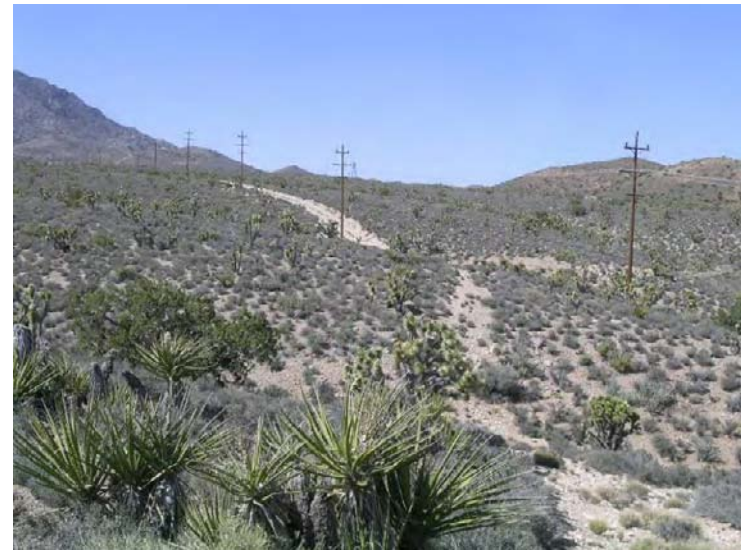
Photograph 12. Looking north along the right-of-way for the Nipton 33kV transmission line.
