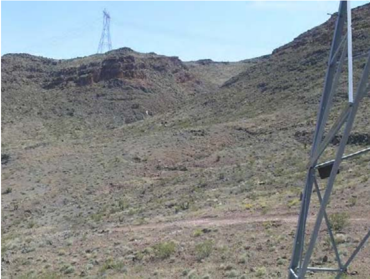
Photograph 5. Looking east from the right-of-way in the McCullough Mountains.
