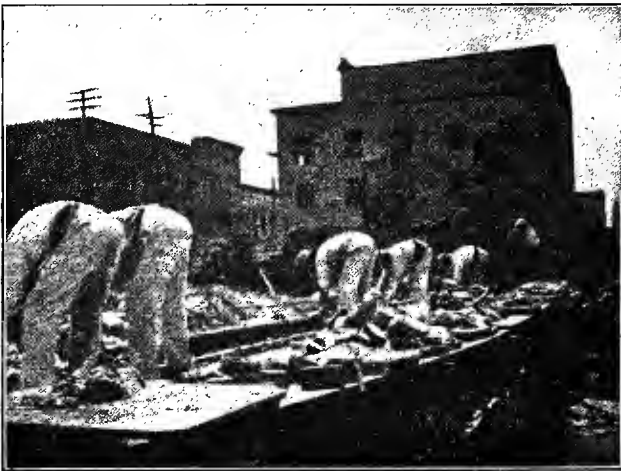
Fig. 303. Bricklayers working in a bent position.
