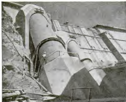
Migrating fish have small chance for life in churning water within these giant penstocks of Shasta Dam
