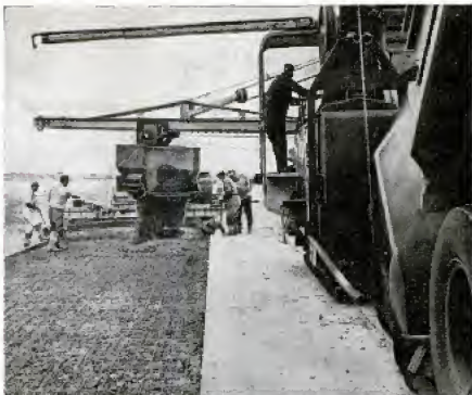
Mixing machine drops concrete on one of six major runways at Idlewild Airport. Below, plans for the 4000-acre landing field and buildings
