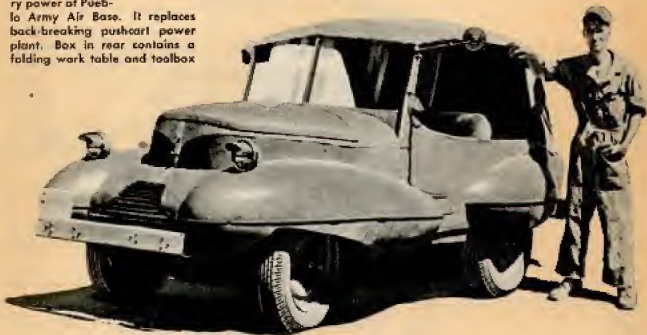
Those teardrop fenders were made from belly tanks of a P-38 and the front grill was part of ammunition rack on a B-24. T/Sgt. Wayne K. Pike of Pittsburg, Kans., stands beside his transformed jeep at a 13th Army Air Force base
