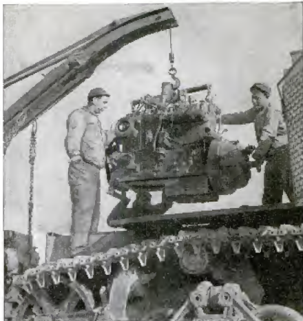
The job of repairing a tank is speeded up by installing a rebuilt engine
