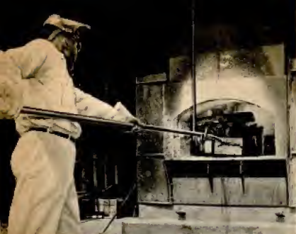
Above, left, parts from wrecked warplanes are pushed into a melting furnace to be reduced to molten aluminum. Right, after "cooking," the aluminum comes out in ingots. Below, left, ultraviolet lamp from a bomber is attached to a base for classroom work. Right, checking spark plugs from old Navy planes for possible reuse
