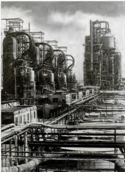
Above, cat crackers dominate scene at Standard Oil's Baton Rouge plant
