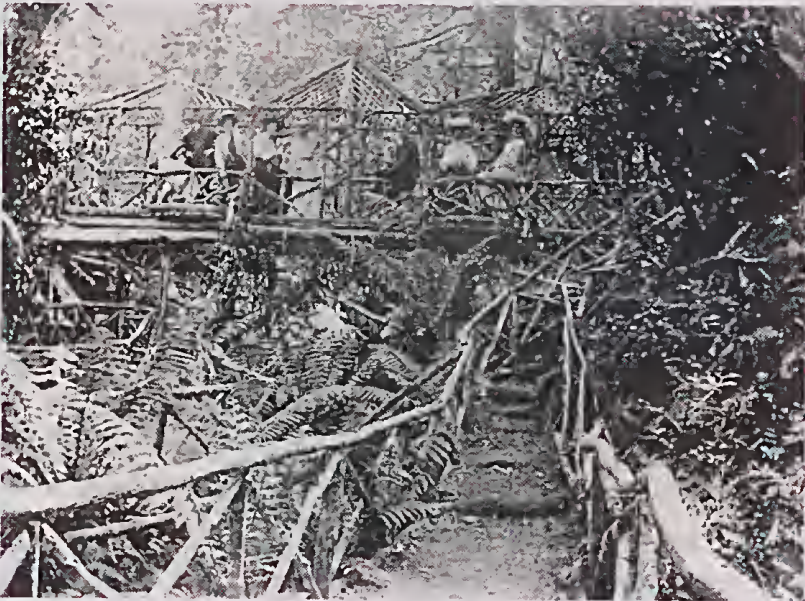
Figure 2. The bridge at the Clematis and Falls hut exemplifies a certain elegance in late 19th Century design.
