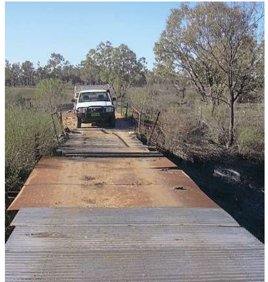
Would you trust your rented BMW to a bridge of sheet steel, corrugated iron and old railway sleepers?
