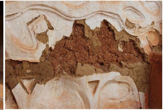
② Decorative elements are also impacted by erosion at the wall base level.
