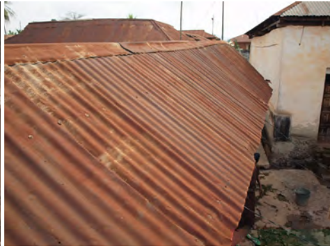
① Roof eaves are too short and do not protect decorative elements. Several sheets are leaking.
