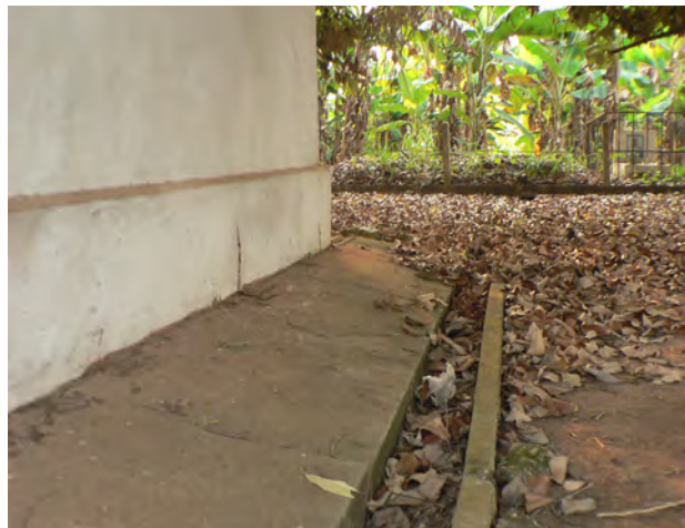
Drainage Channel at Asenemaso
