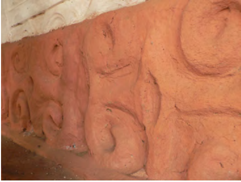
① Inconsistent and poor repairs to decorative elements.
