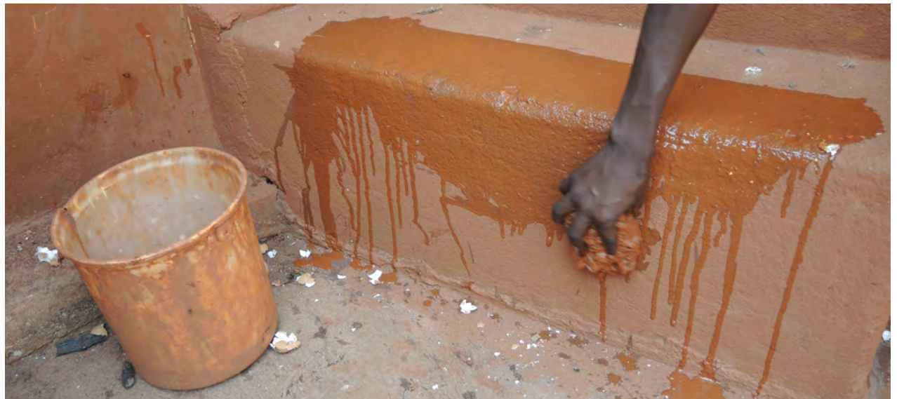
Red Clay Slurry Application at Abirim
