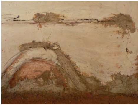
① Inconsistent and poor repairs to decorative elements.
