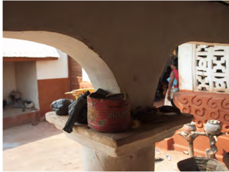
① Custodians have restored the rooms around the courtyard without respect to material authenticity. Concrete columns replaced original thick mud posts, but the Shrine Building itself has remained untouched.
