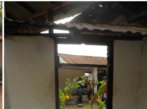
④ The roof is in poor condition, many parts are leaking.
