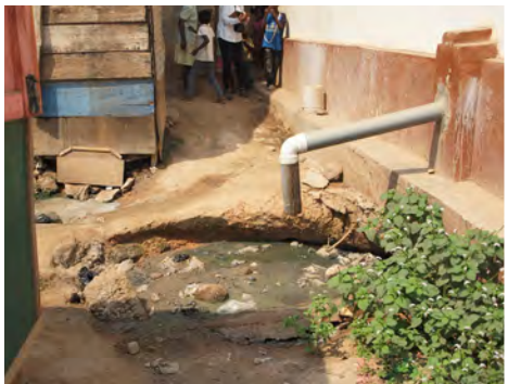
④ Soak away pit chocked on the southern side, behind the kitchen.
