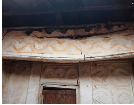
① Collapse is imminent in many places within the interior.
