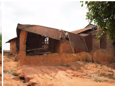
④ The roofs and walls of the Chief's Palace complex are in a very poor state. Many elements have collapsed already. The central room where the chief sits is the last standing element.
