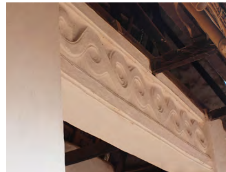
⑦ The walls are well maintained and regularly repainted.
