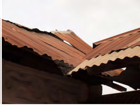
① The roofing sheets are aging and the roof is leaking. Some of the sheets could easily be removed in a severe storm.
