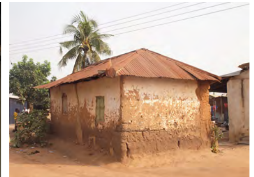
⑤ The walls are in poor condition due to the roof leakages and short overhangs.
