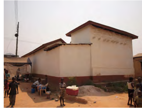
② Room added to anterior, between the Drummers' Room and the Shrine Room without GMMB's consent. However, it cannot be seen from the Courtyard.
