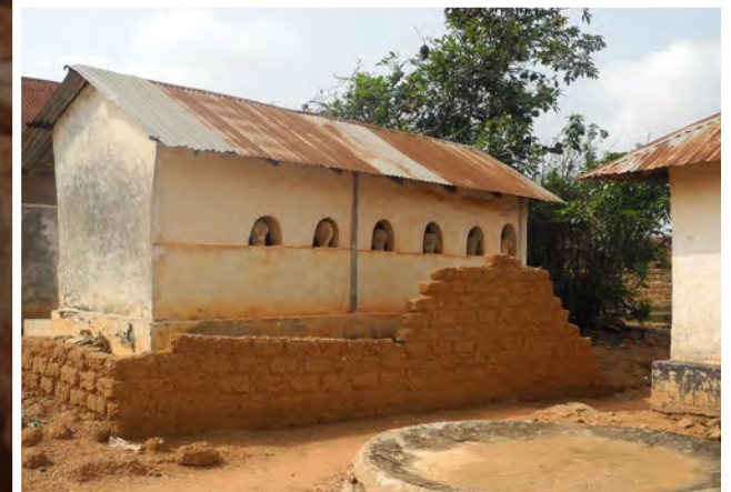
Mausoleum Exterior at Patakro
