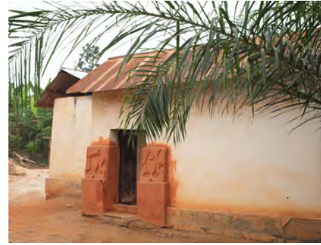
③ The structure is sound.
