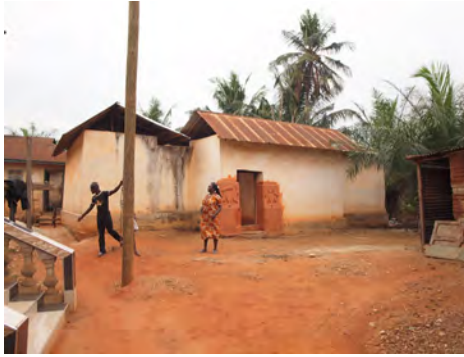
① The site is clean and rather well kept.
