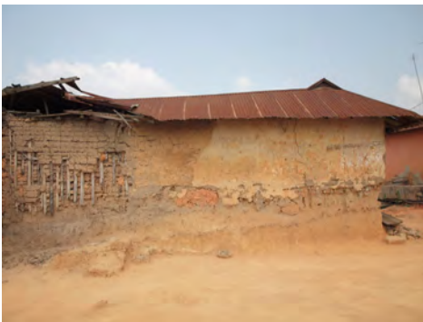
④ The roofs and walls of the Chief's Palace complex are in a very poor state. Many elements have collapsed already. The central room where the chief sits is the last standing element.
