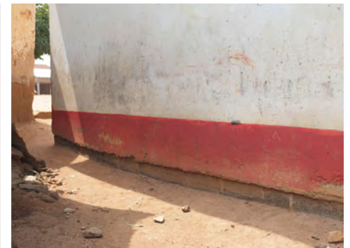
⑥ Industrial red paint has been introduced instead of the traditional red ochre wash.
