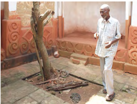
④ The courtyard is covered with cement slabs that prevent the ground from drying.
