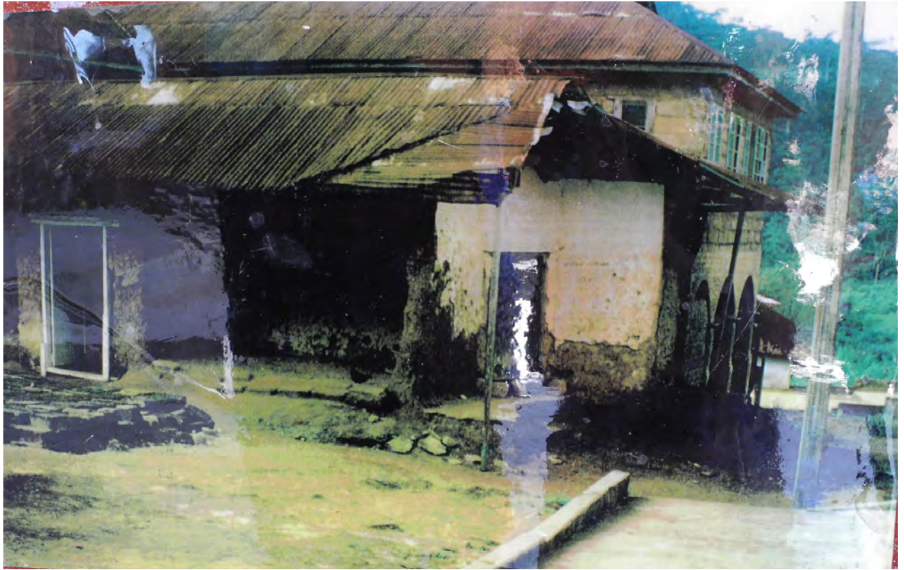
Photograph of Demolished Shrine at Obomeng
