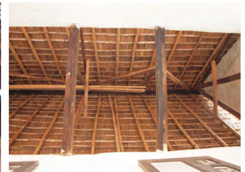
⑧ The bamboo roof structure resists termites.
