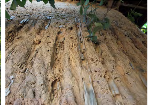
③ In particular, the anterior wall of the reception hall is highly eroded.
