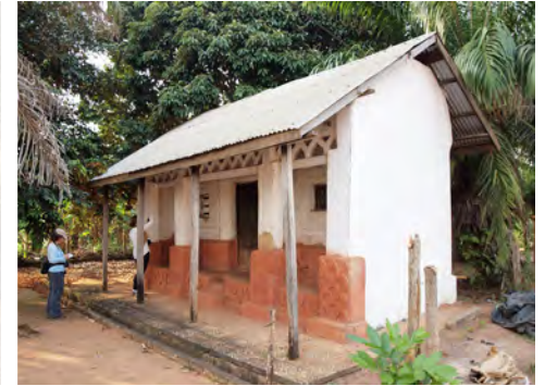
④ The roof is well conserved.
