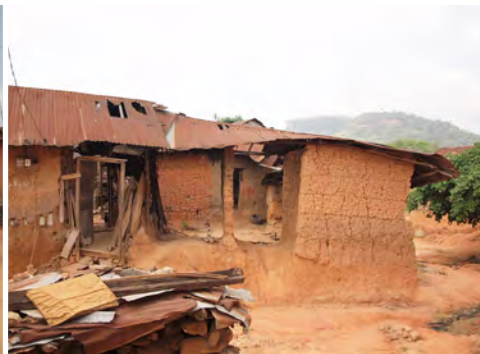
④ The roofs and walls of the Chief's Palace complex are in a very poor state. Many elements have collapsed already. The central room where the chief sits is the last standing element.
