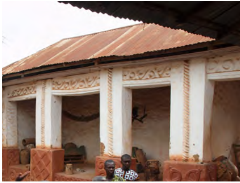
① Roof eaves are too short and do not protect decorative elements. Several sheets are leaking.
