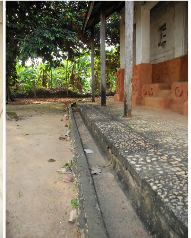
Drainage Channel at Asenemaso
