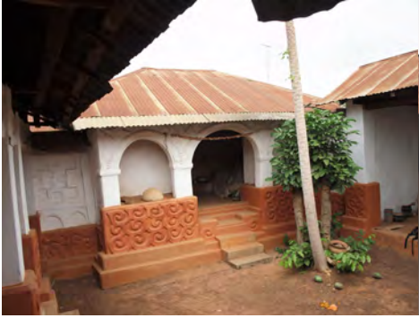
① The roofing sheets are aging and the roof is leaking. Some of the sheets could easily be removed in a severe storm.
