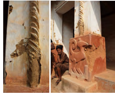
② Decorative elements are also impacted by erosion at the wall base level.
