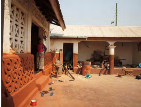
① Custodians have restored the rooms around the courtyard without respect to material authenticity. Concrete columns replaced original thick mud posts, but the Shrine Building itself has remained untouched.
