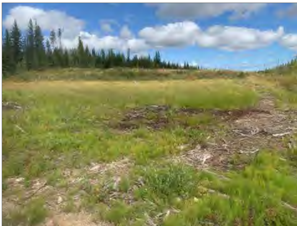
Plate 3.3-3. Modified portion of a Wb06 Tamarack - Water sedge - Fen moss bog at Plot WL226 showing the cleared transmission line and construction road.
