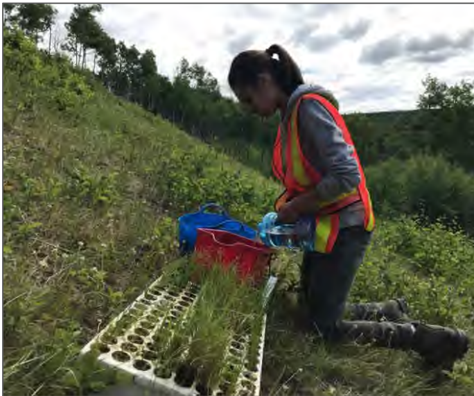
Plate 3.3-3 Local technician preparing the soils and water mix to place within the excavated hole along with the plant.
