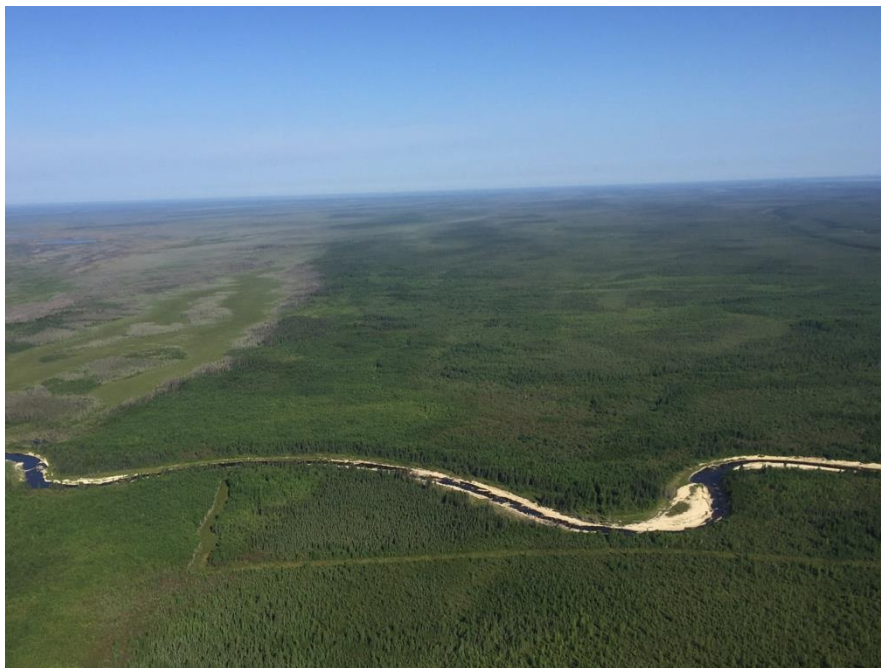
Photo 9: Aerial view of Buffalo Creek, looking west at where the Reach 2 berm is proposed to be constructed (taken on August 03, 2016)
