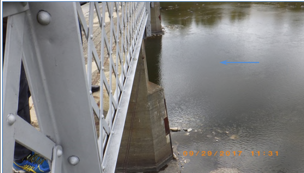
Upstream side of existing bridge pier – Canadian side
