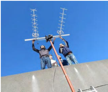
Figure 4: UHF Antenna being set up at Miguelete campus
