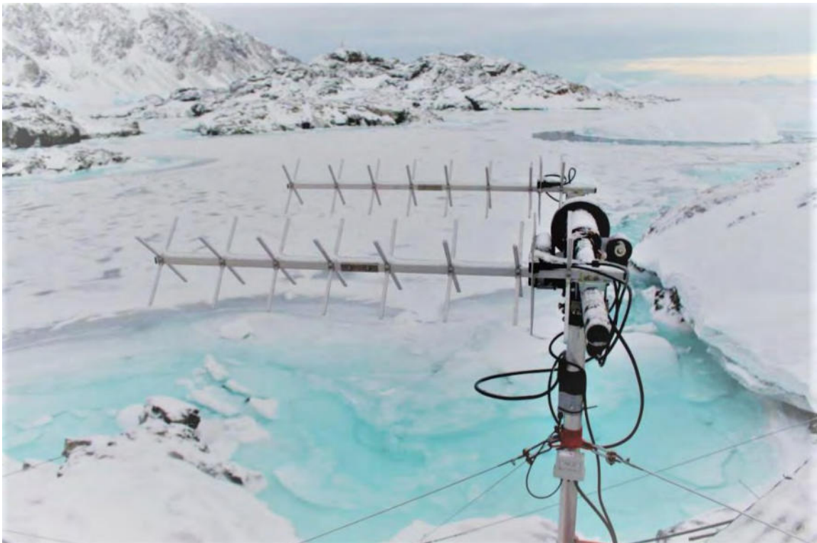
Figure 8: Fully installed antenna in the Antarctic Ground Station (as of June 2019)
