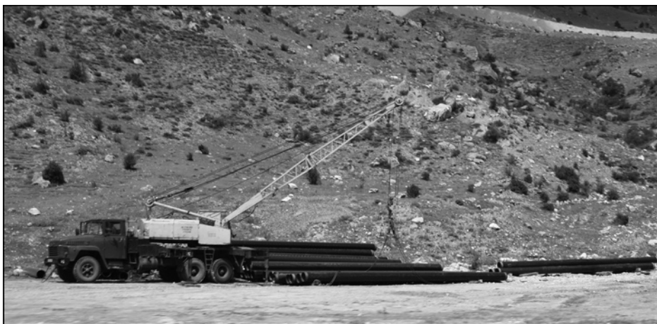
Fig. 5. Unloading of pipe in North Ossetia for construction of the Alagir–Tskhinvali natural gas pipeline. Photograph by the author, August 2008.
